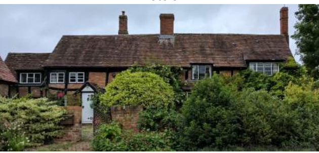
Photo 3 Front South Facing Elevation
