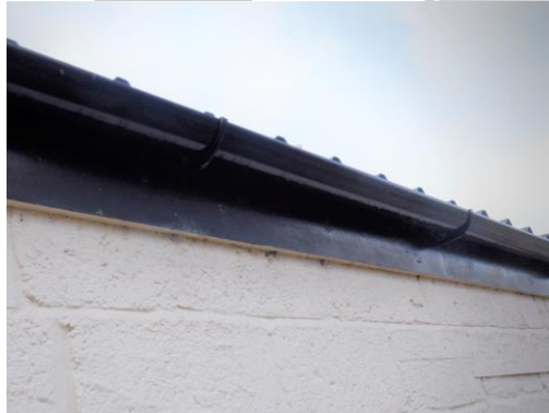
FIGURE 11: THE GARAGE BARGEBOARDS.
