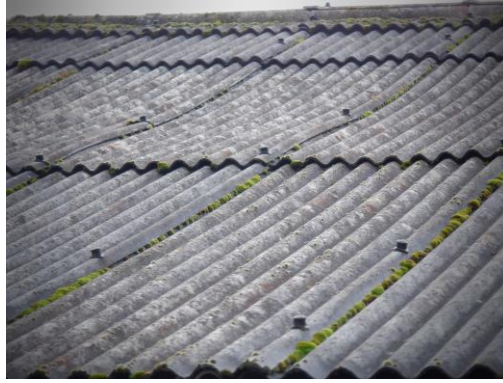
FIGURE 9: THE ASBESTOS / CONCRETE FIBRE ROOF OF THE BARN.
