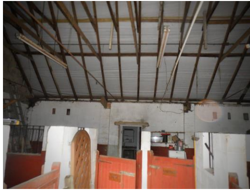
FIGURE 5: ROOM 1 SHOWING THE INSIDE OF THE ROOF.
