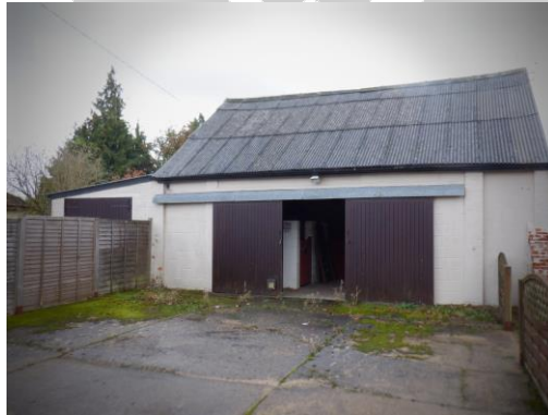
FIGURE 3: A VIEW OF THE BARN FROM THE NORTH.
