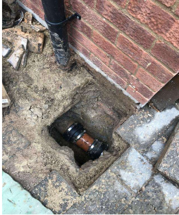
T/H1 - Repair to Run 7 following survey
