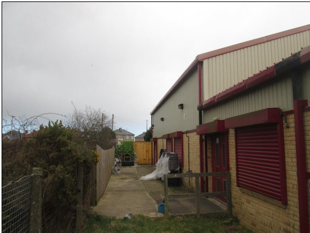
Rear elevation of community centre.
