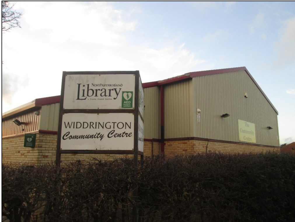
Side elevation of community centre from Grange Road.
