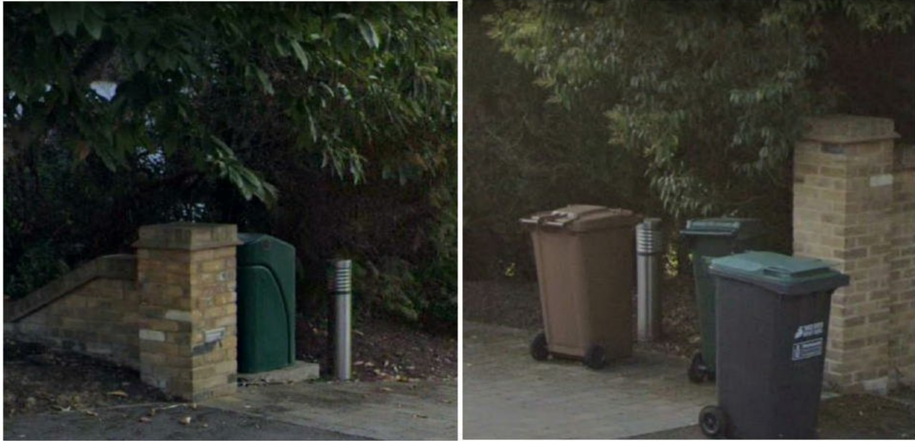
Figure 1. Lighting columns at 43 Astons Road
