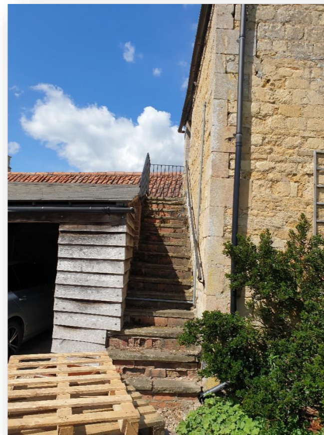
View of existing external steps to the 1 st floor
