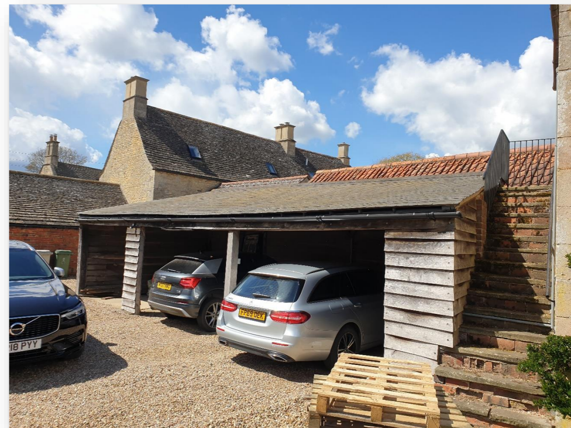
View of the existing car port looking west towards No.10 Main Street
