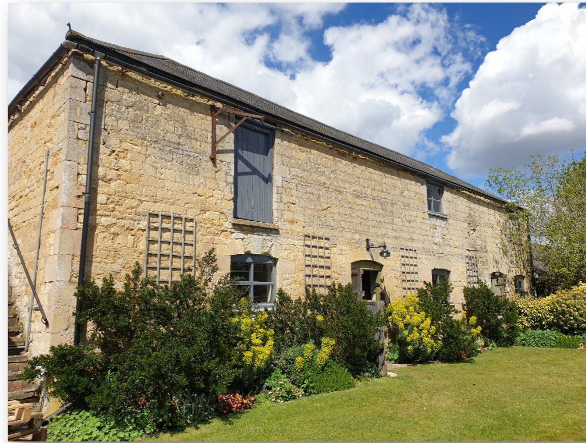
Frontage of barn viewed from the driveway
