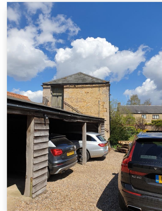
Side view of the barn from the driveway
