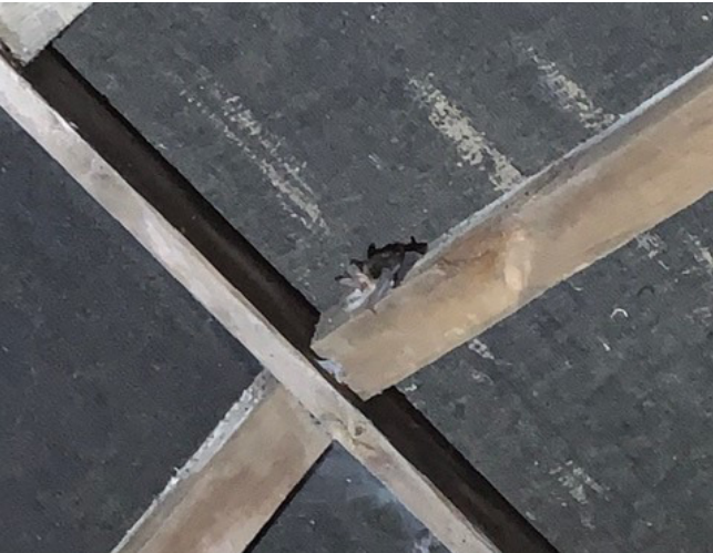
BLE within building interior
