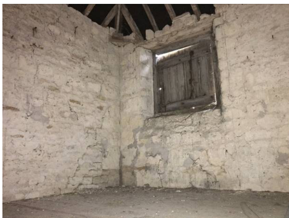
First floor room east end
