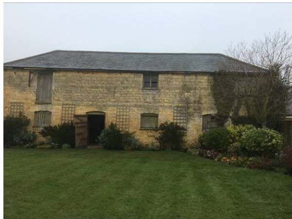
Front of building
