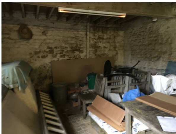
Ground floor storage room
