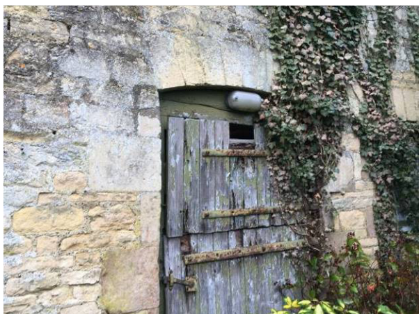
Door to room at eastern end of building
