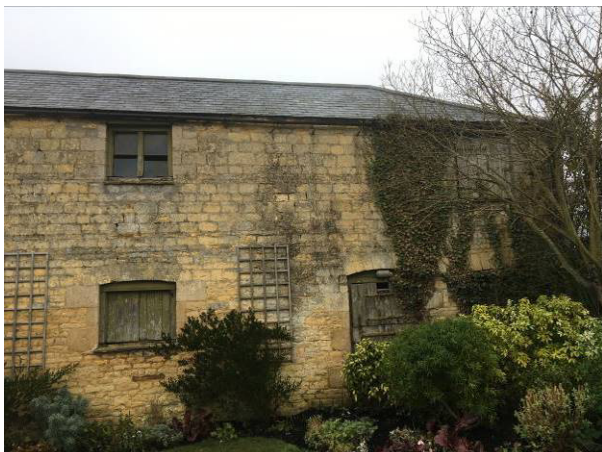
Close up of east side
