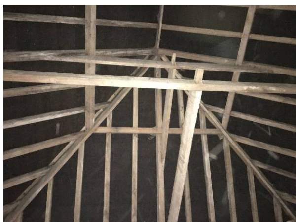
Underside of roof at eastern gable
