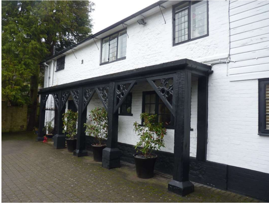
Existing front elevation of Old Rosings
