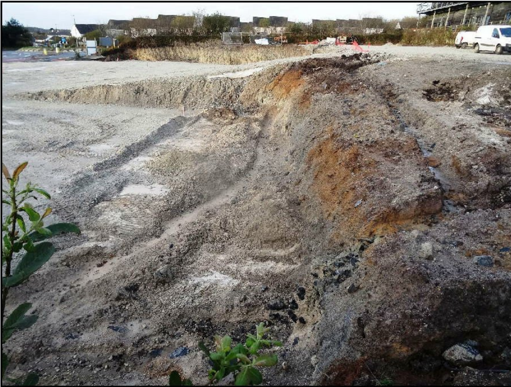
Fig 2: Footings, looking west.
