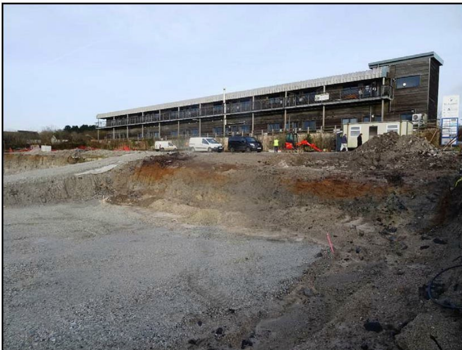
Fig 1: Footings, looking north-west.
