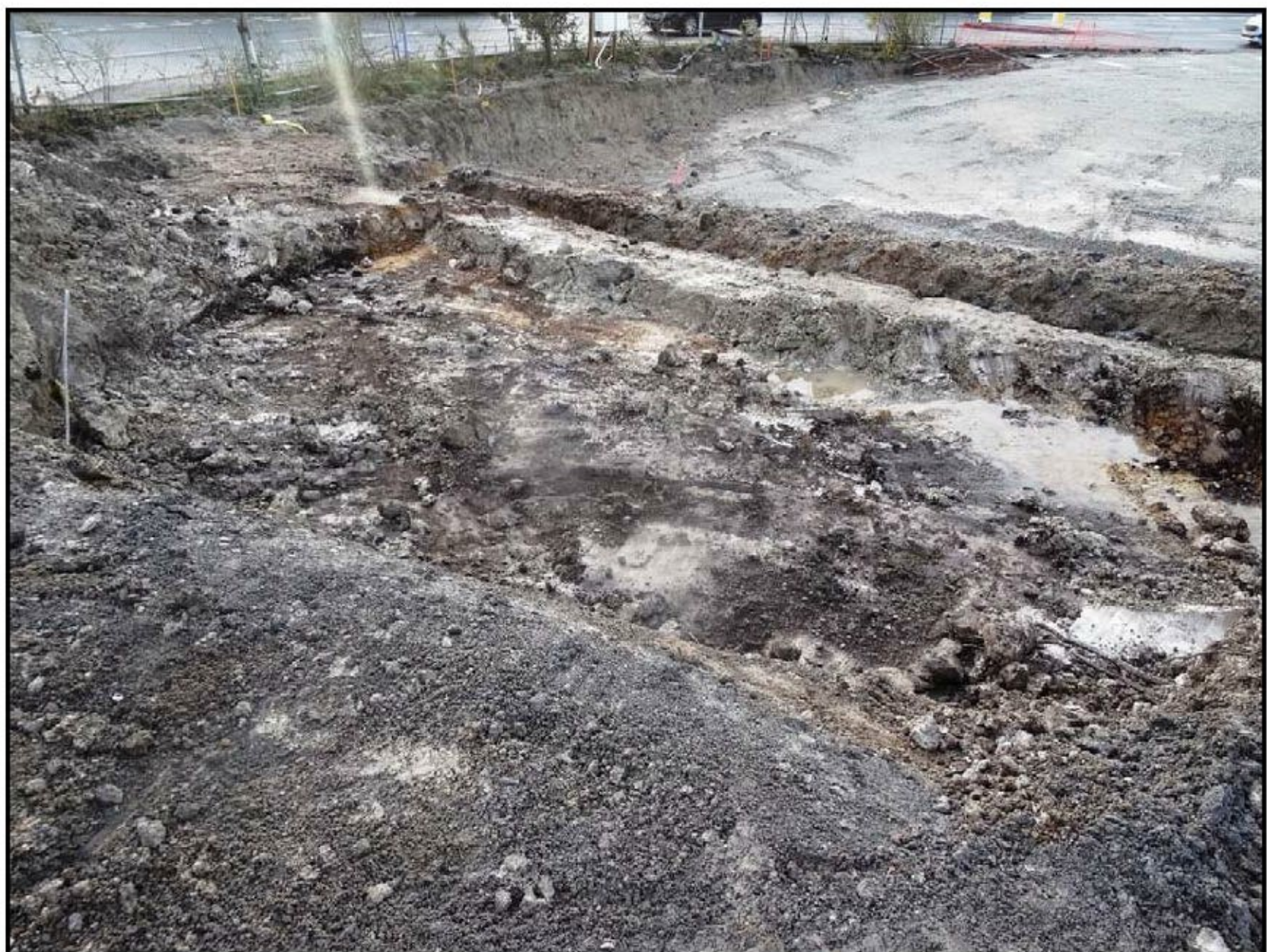
Fig 3: Footings, looking south-east.
