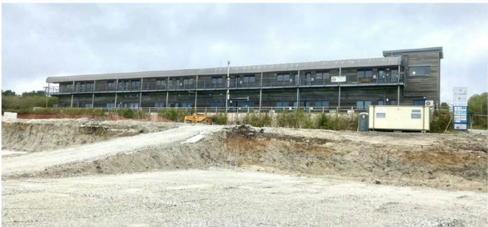
Two storey building to north
