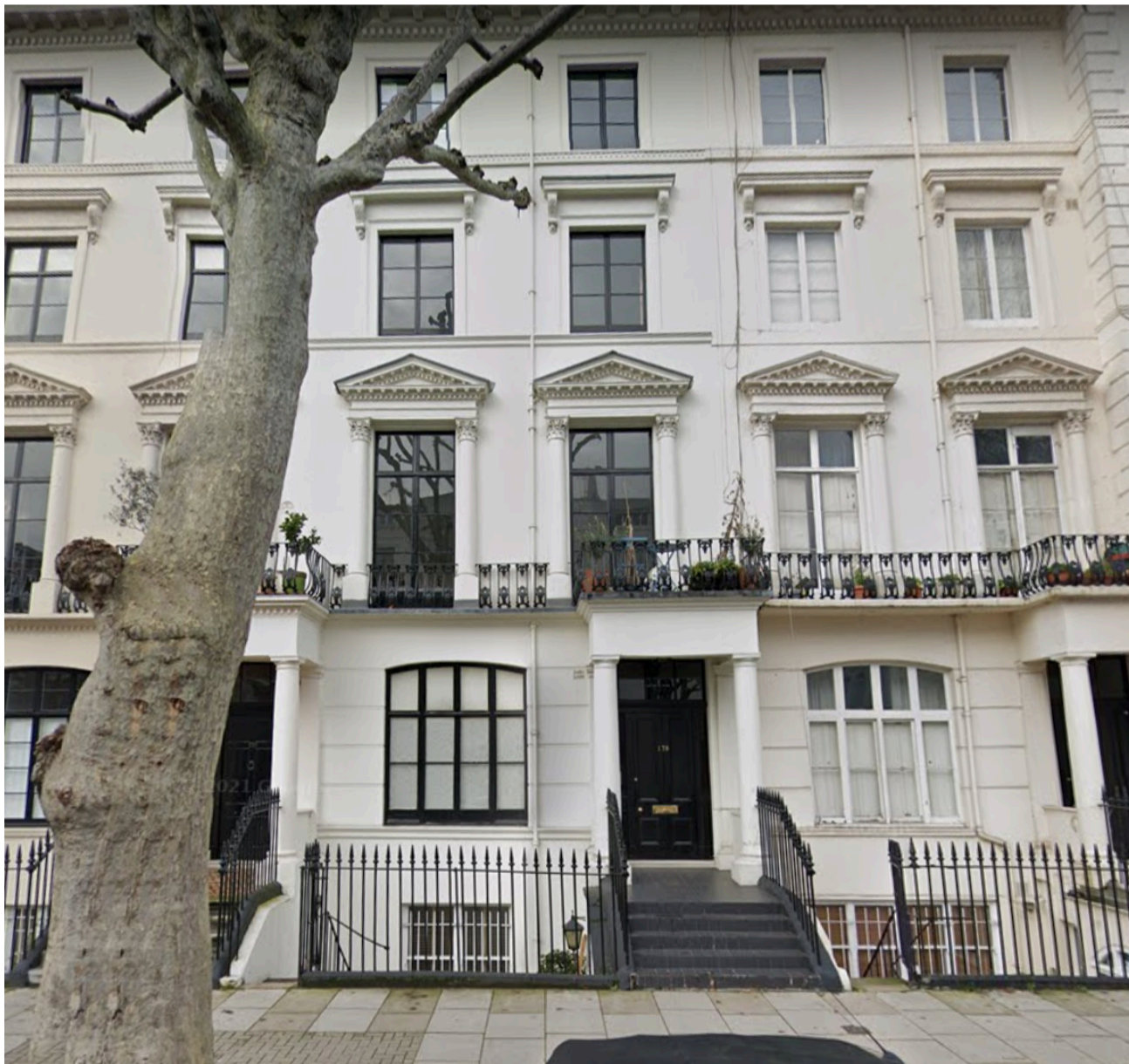
Photograph from Sutherland Avenue
