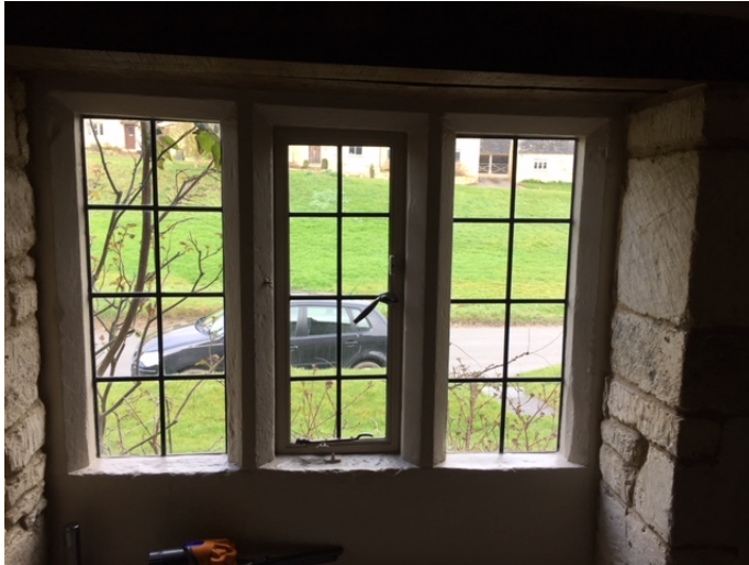
Photos 4 & 5: showing one of the mullion window casements from inside and the centre casement opens
