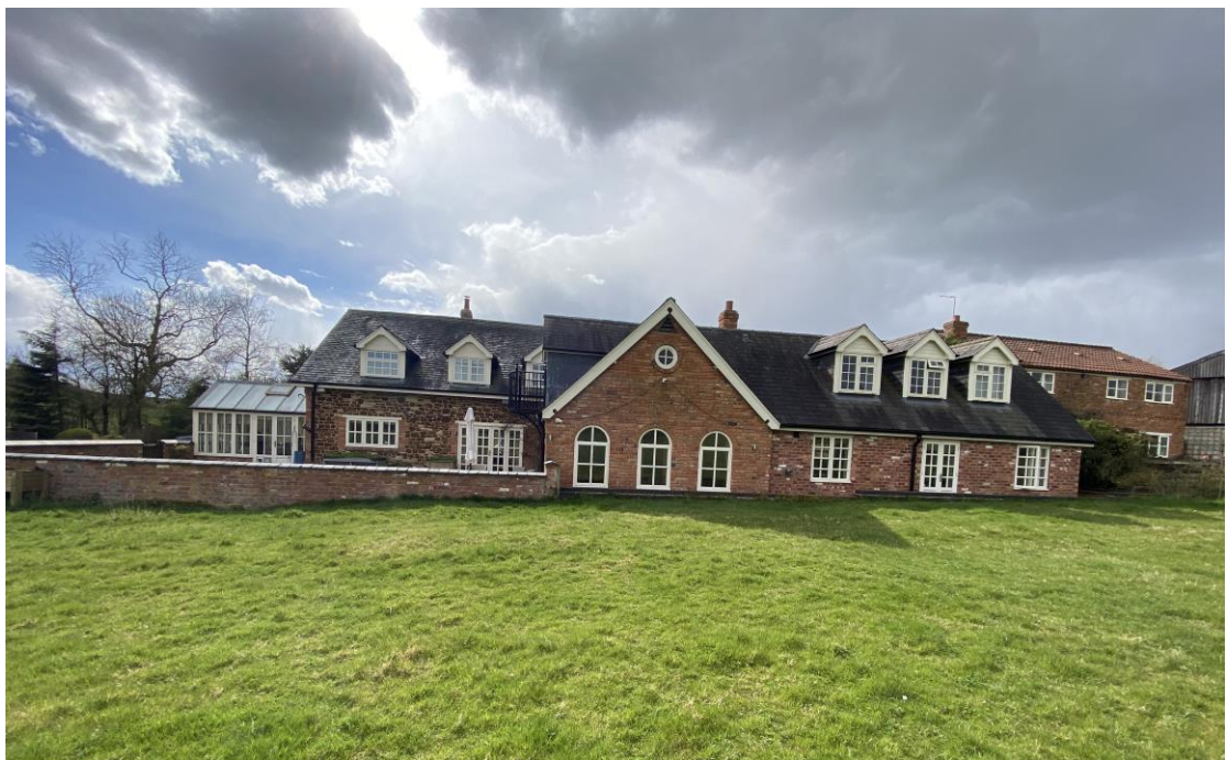
Above photos – photos of the rear elevation of the existing property (part and full images).
