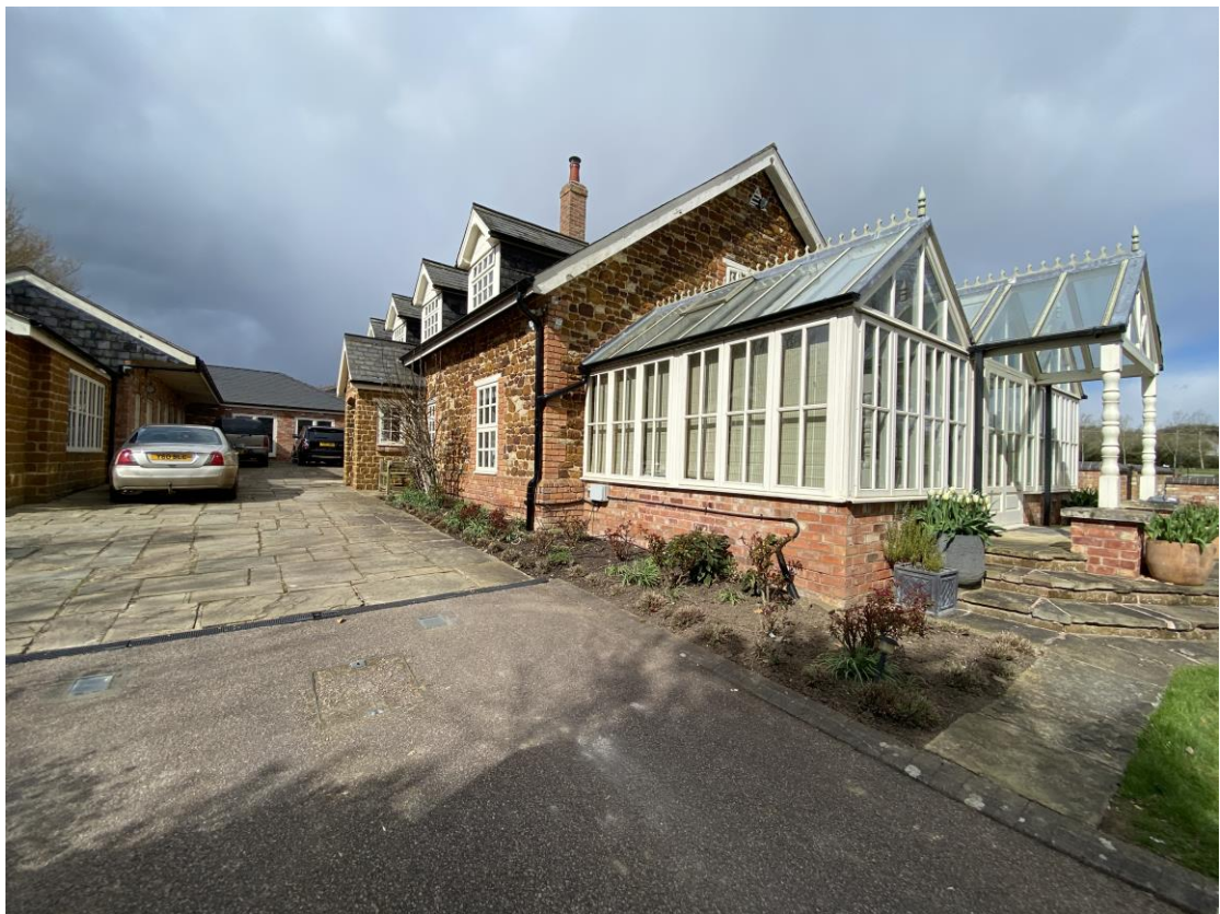
Above photo – existing glazed garden room structure.
