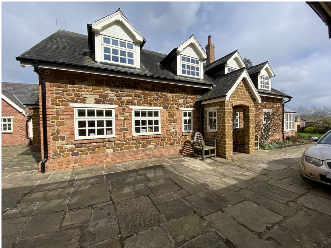
Above photo – part of existing property’s front elevation.
