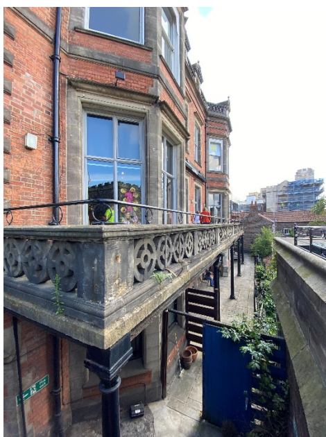
IMG_1902 Existing external balcony seating area
