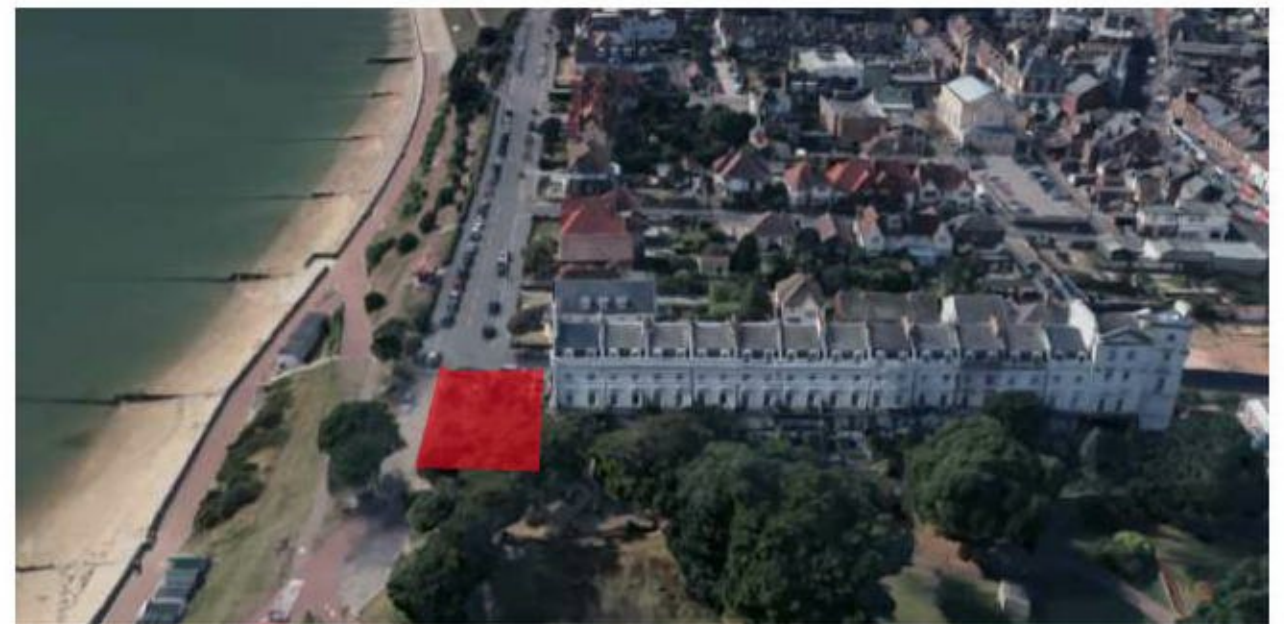
Figure 39 – Birds eye view of Orwell Terrace from Cliff Park. The application site is marked in red.
