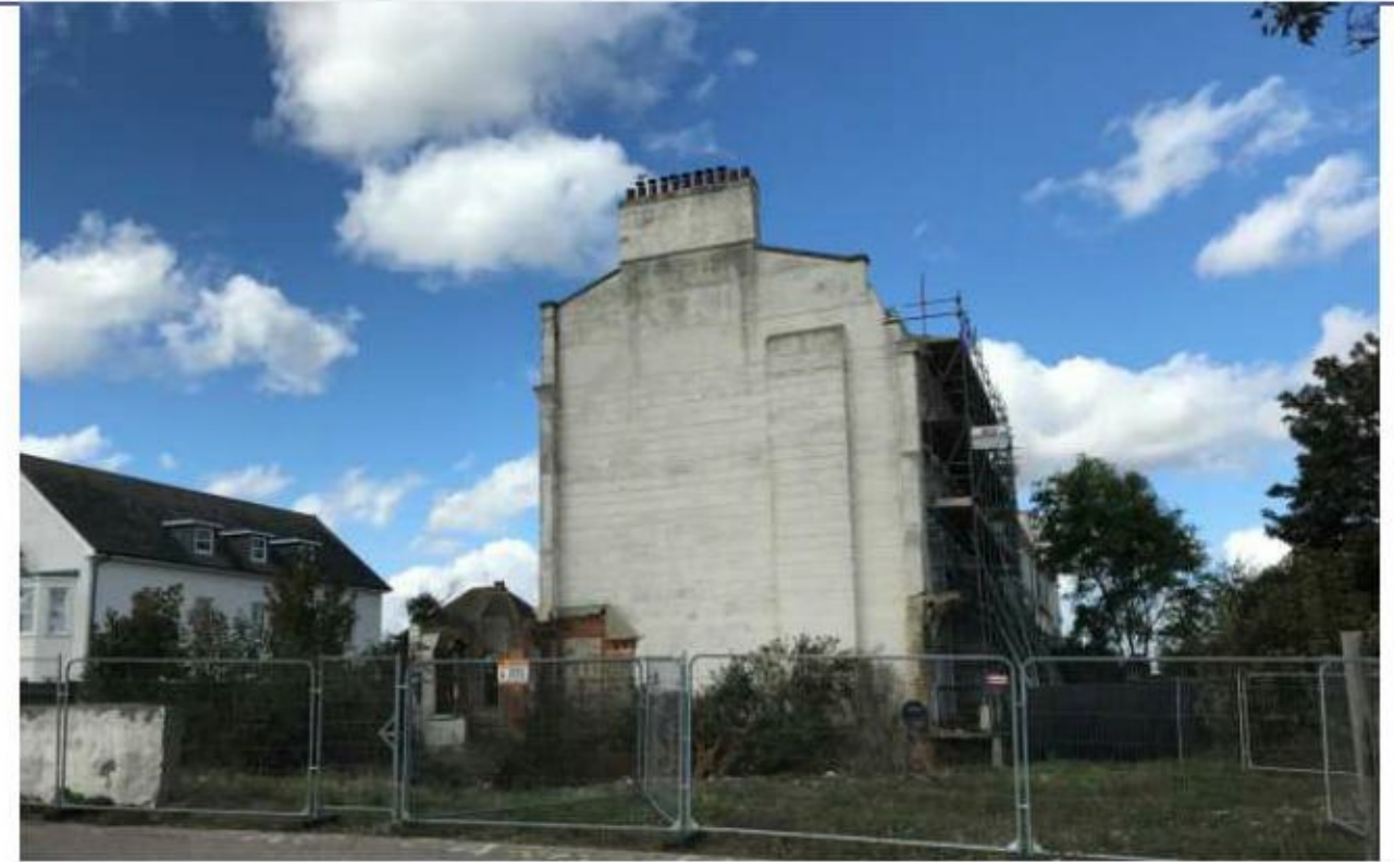
Figure 43 – View of the side elevation
