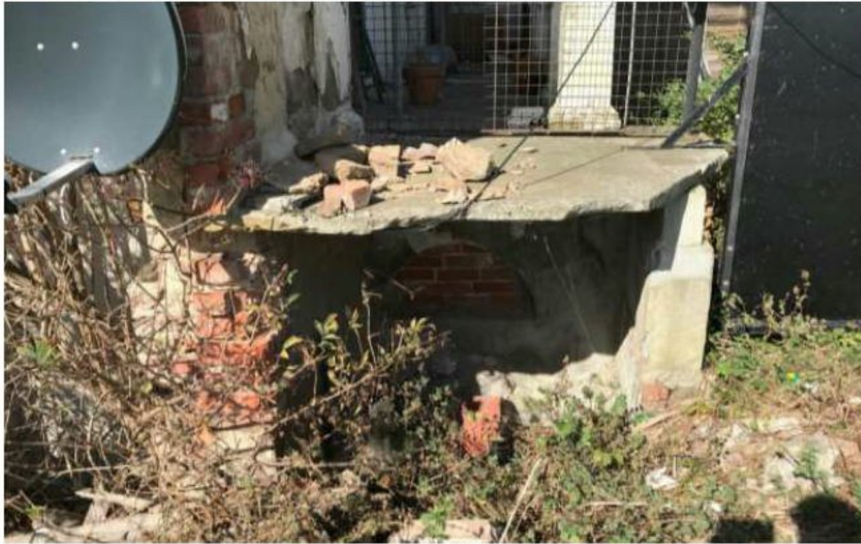
Figure 46 – View of the remains of the building
