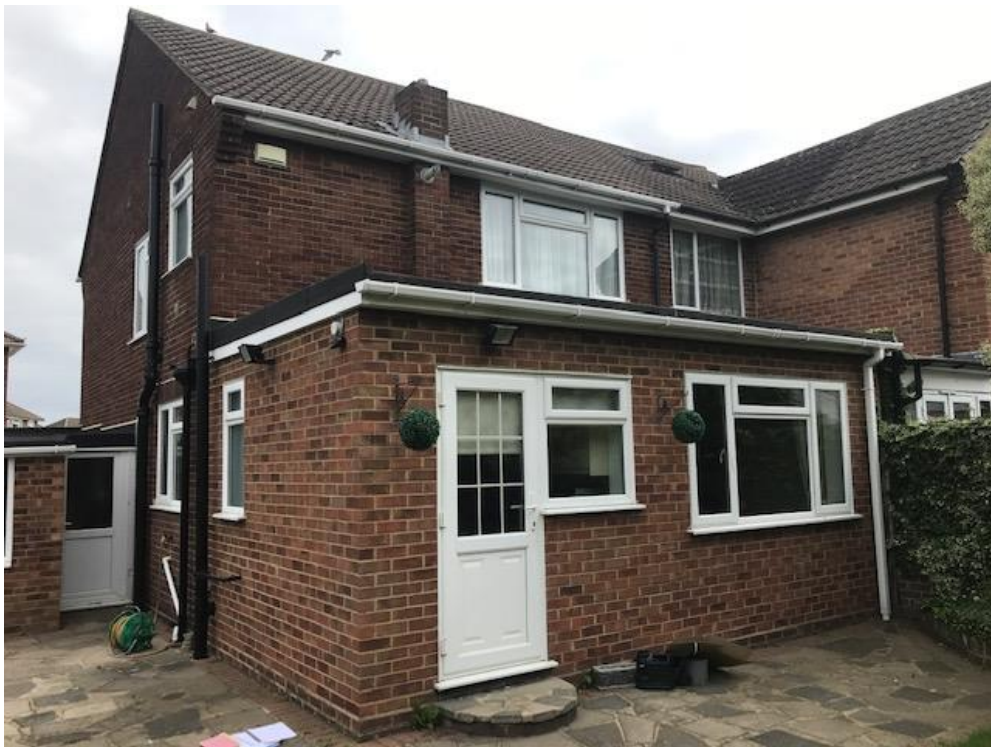
Photo of rear of 12 Stuart Evans Close showing single storey rear extension and rear facing first floor windows set in from flank of property
