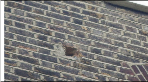
Plate 5: Cavity in brickwork. Part of ventilation apparatus.
