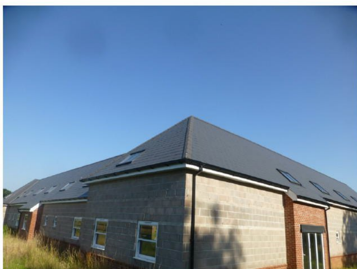
Figure 5. S & W elevations of building
