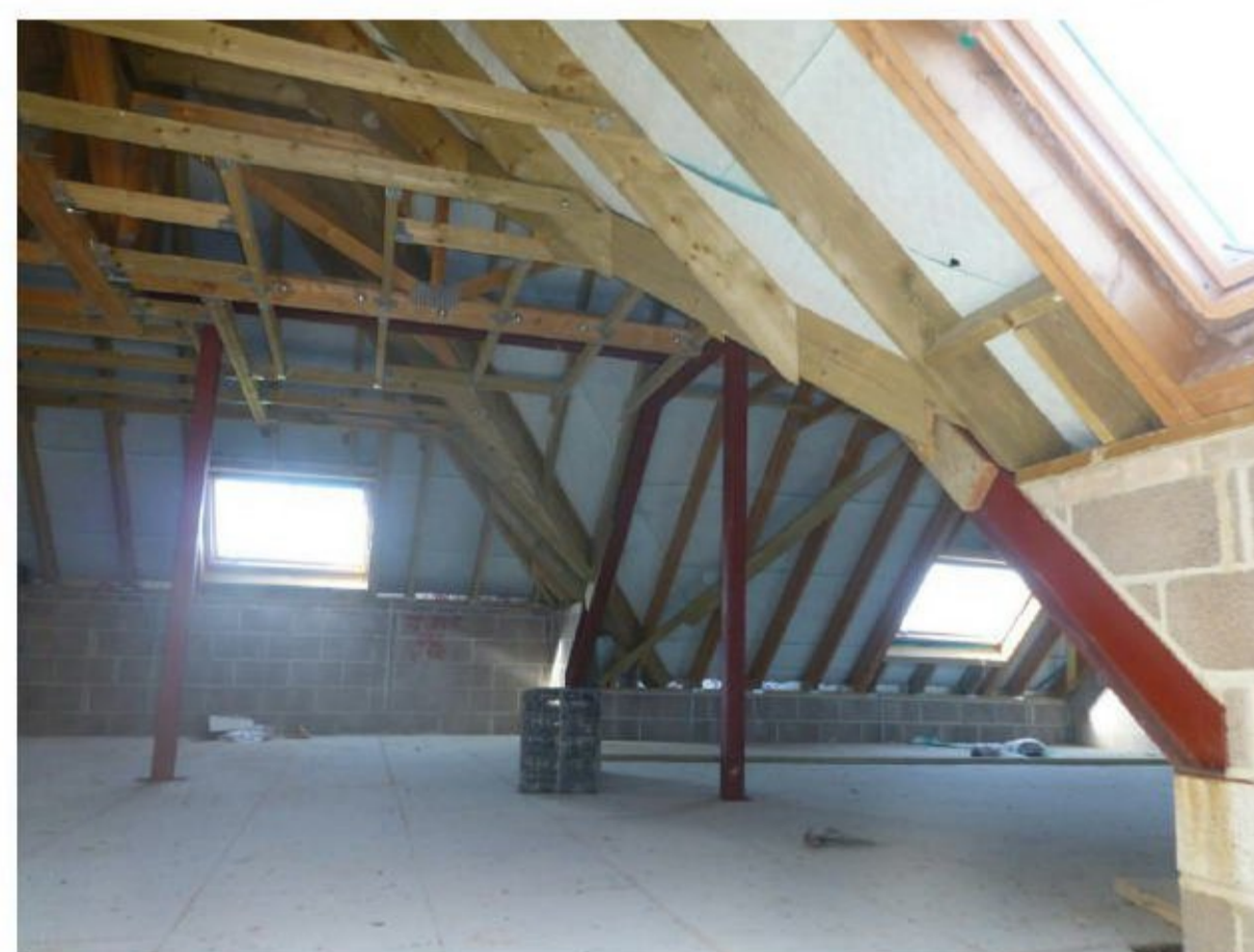
Figure 6. Example of first floor of building
