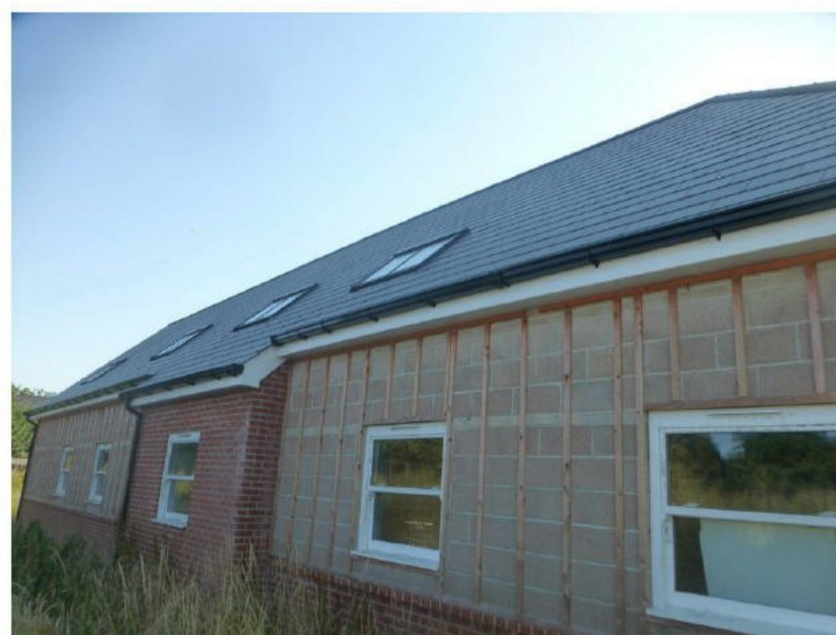
Figure 4. Rear of buildings (S)
