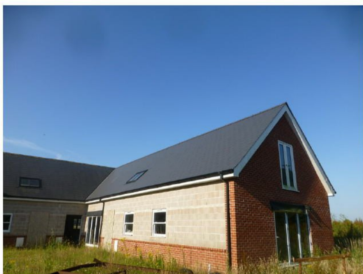
Figure 3. View of building N & E elevations
