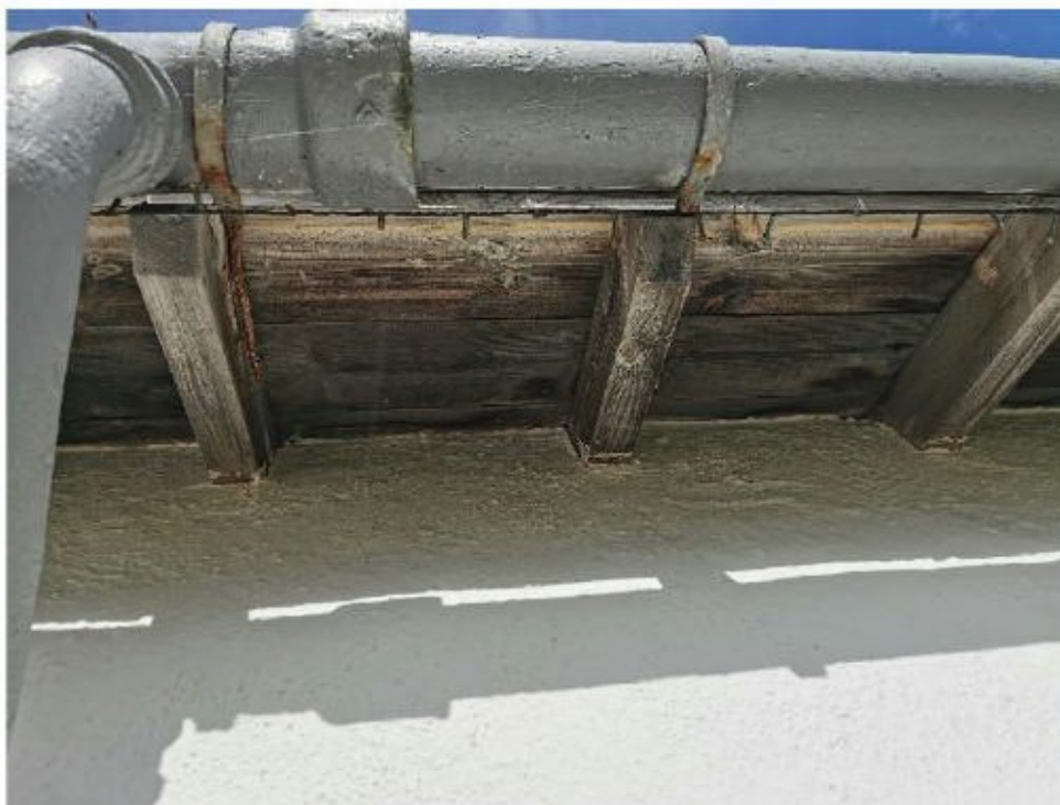
Image 3. Soffits of main building
