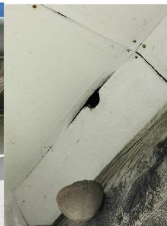
Image 4. Potential entry point towards the west of the building
