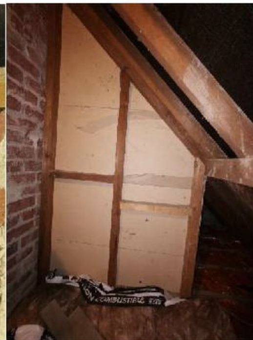
Image 6. Dormer on east side fully inspected
