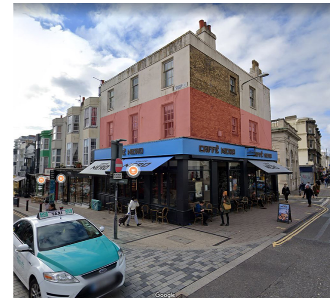
fig. 02- 84 & 85 Western Road- street view with the proposed works area highlighted in red
