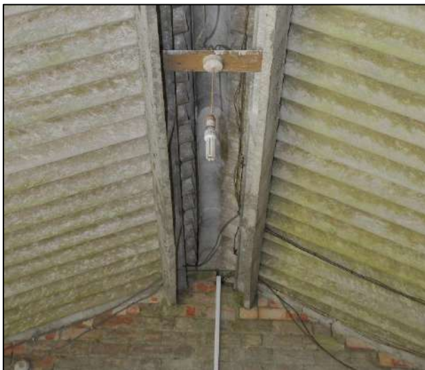
↑ Plate Eleven - Barn Two ridge construction
