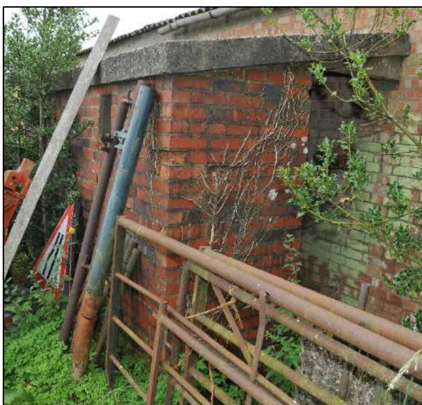
↑ Plate Nine - Barn Two annexe building
