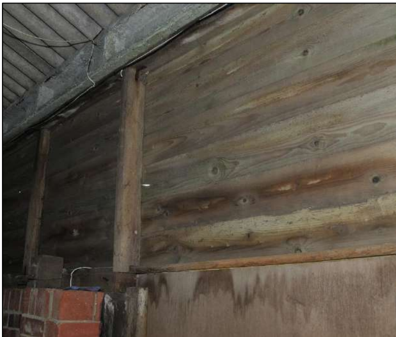
↑ Plate Thirteen - Barn Two interior of weatherboard wall construction
