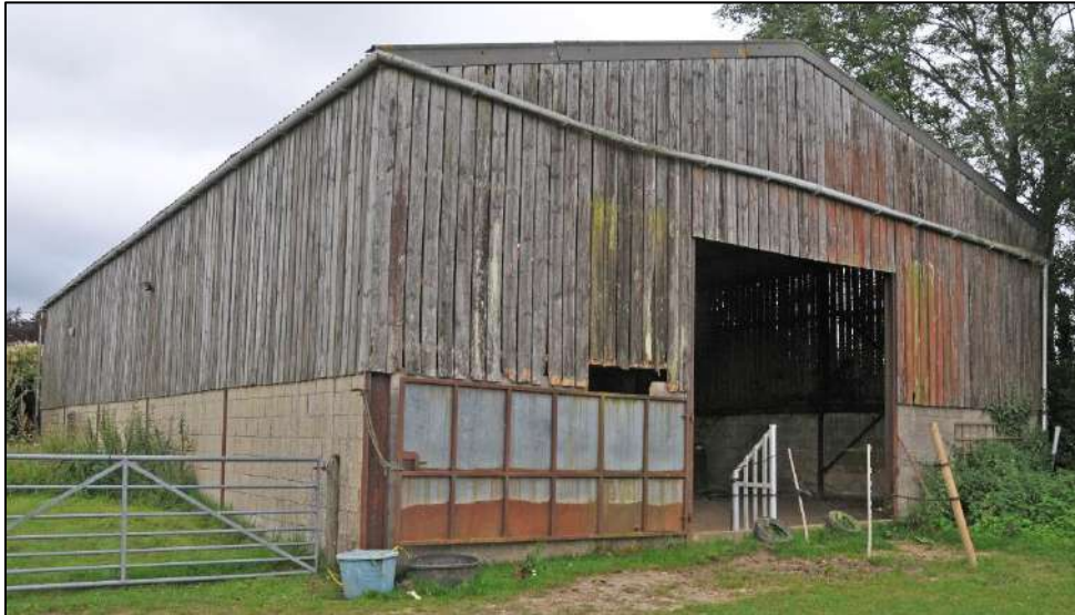
↑ Plate Four - Barn One external character
