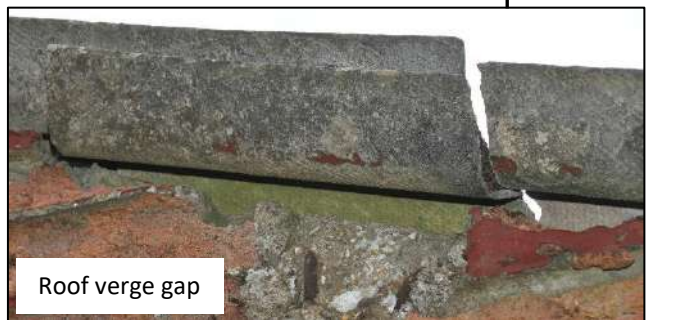
↑ Plate Fifteen - Barn Two West Gable wall potential bat roost features: Dense Ivy growth and roof verge gap
