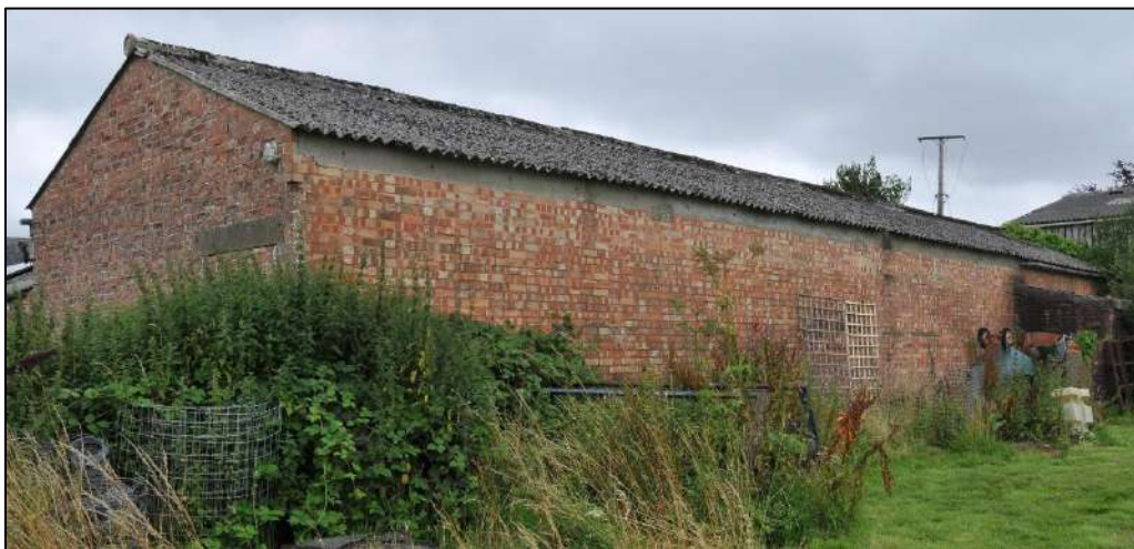
↑ Plate Eight - Barn Two external character
