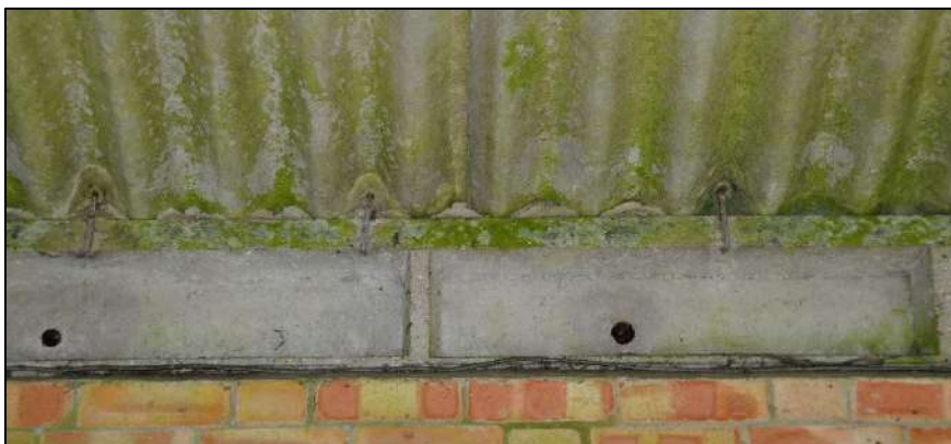
↑ Plate Twelve - Barn Two roof eave construction
