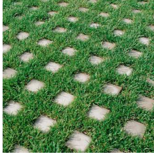
Seeded matrix paving
