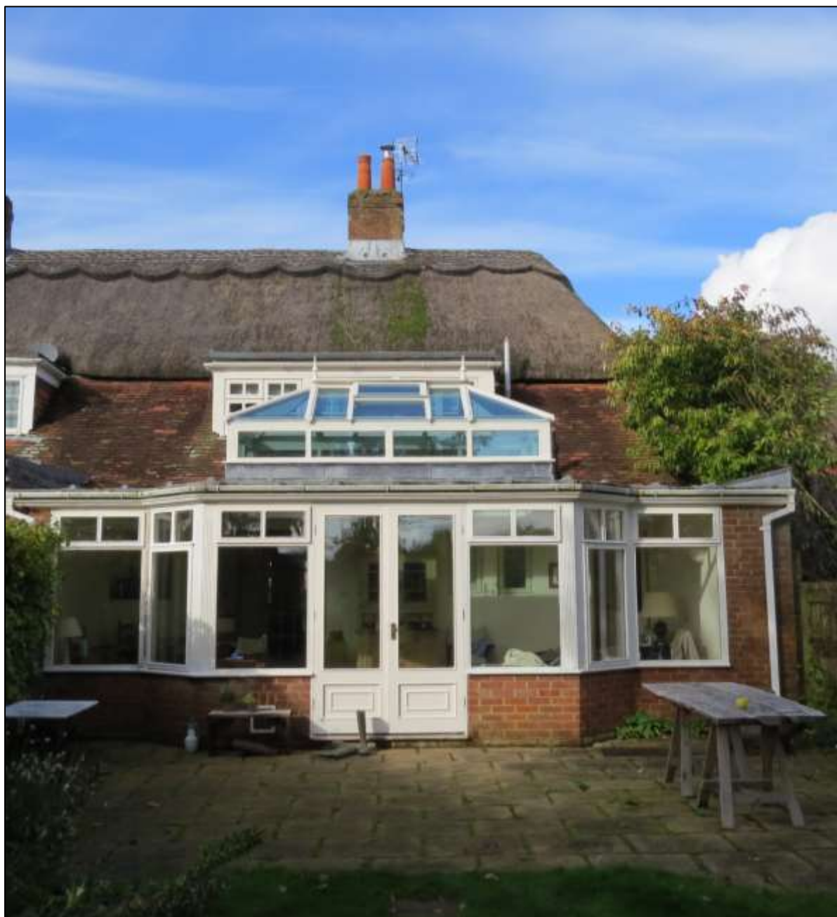
Plate 2 The rear elevation of the property
