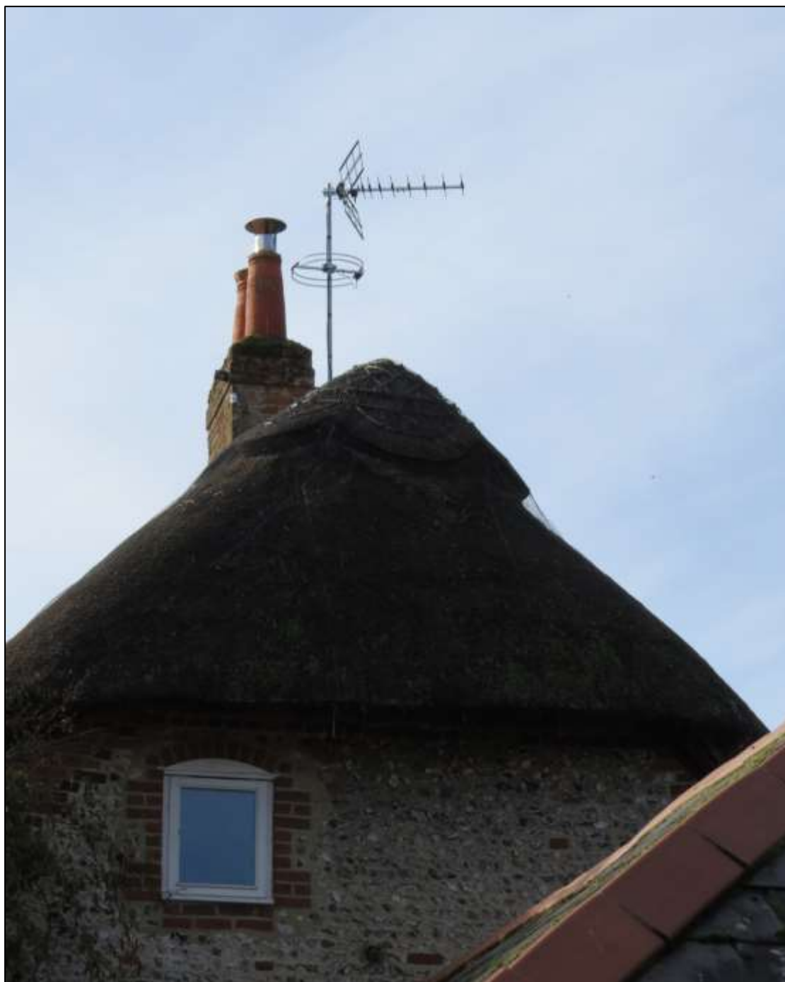
Plate 3 The end elevation of Tichborne Cottage
