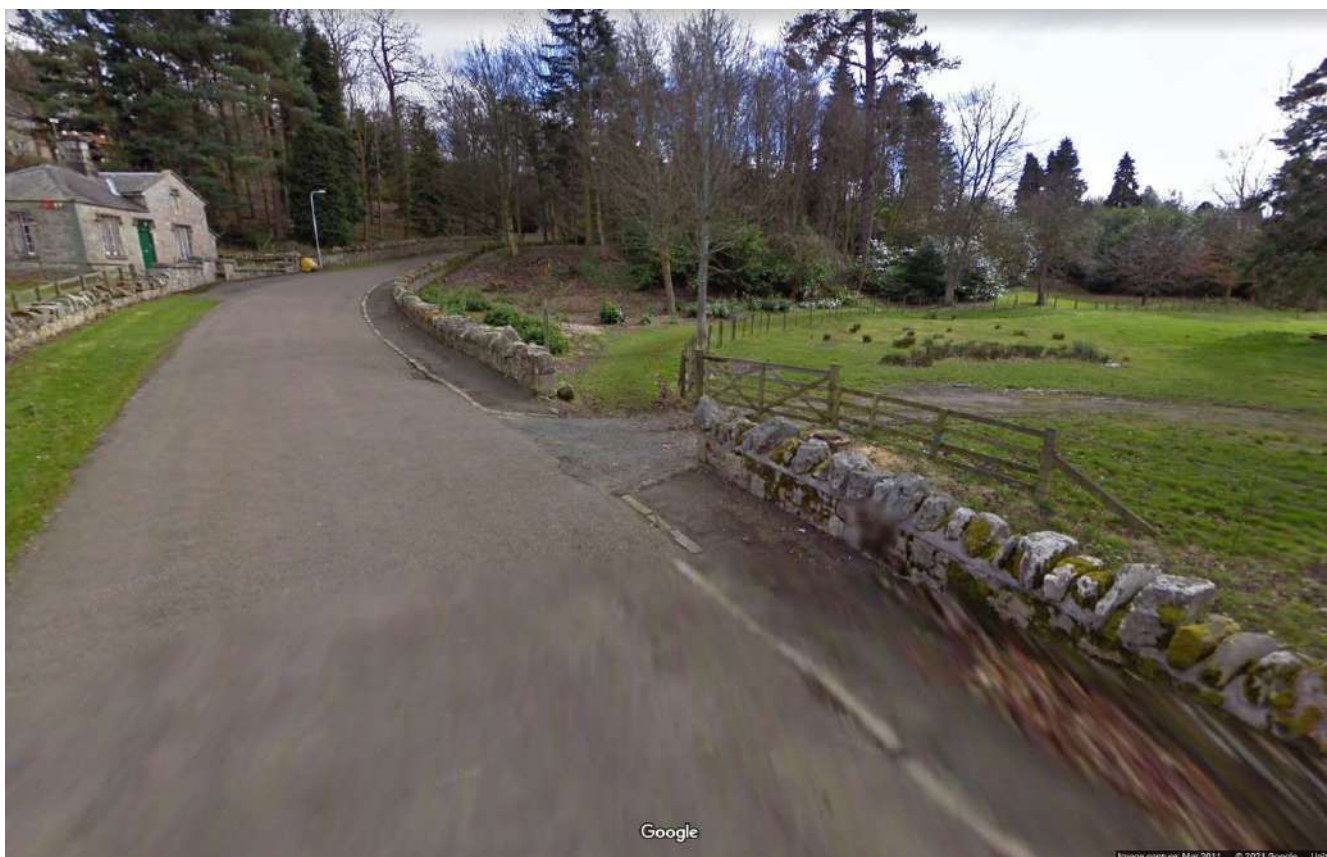
Figure 3-2 Photograph of Field Access (Source: Google Street)
