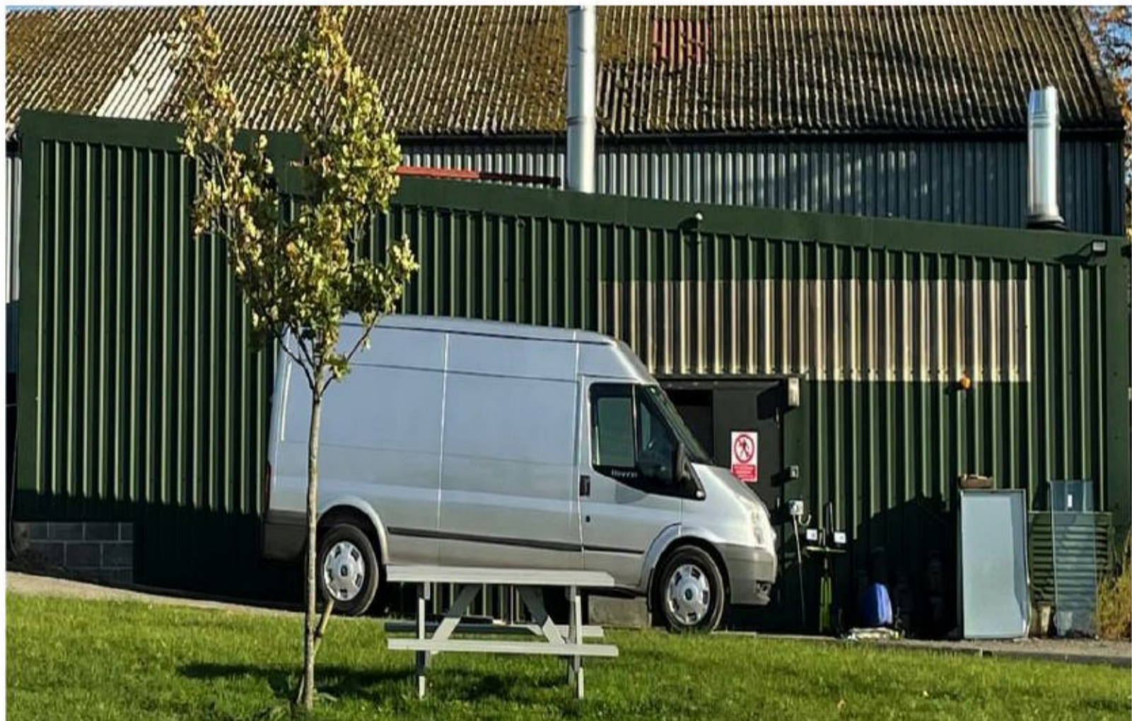
Photograph 7: Attached building - western elevation
