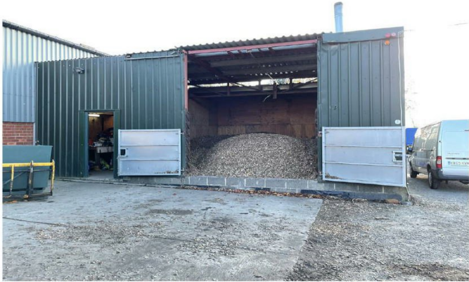
Photograph 6: Attached building - northern elevation
