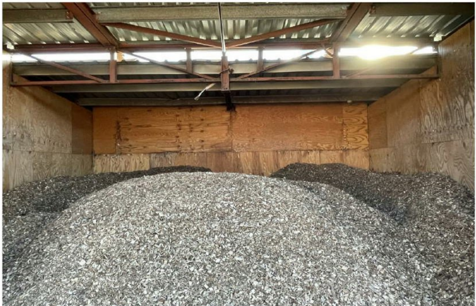
Photograph 9: Attached building - internal view
