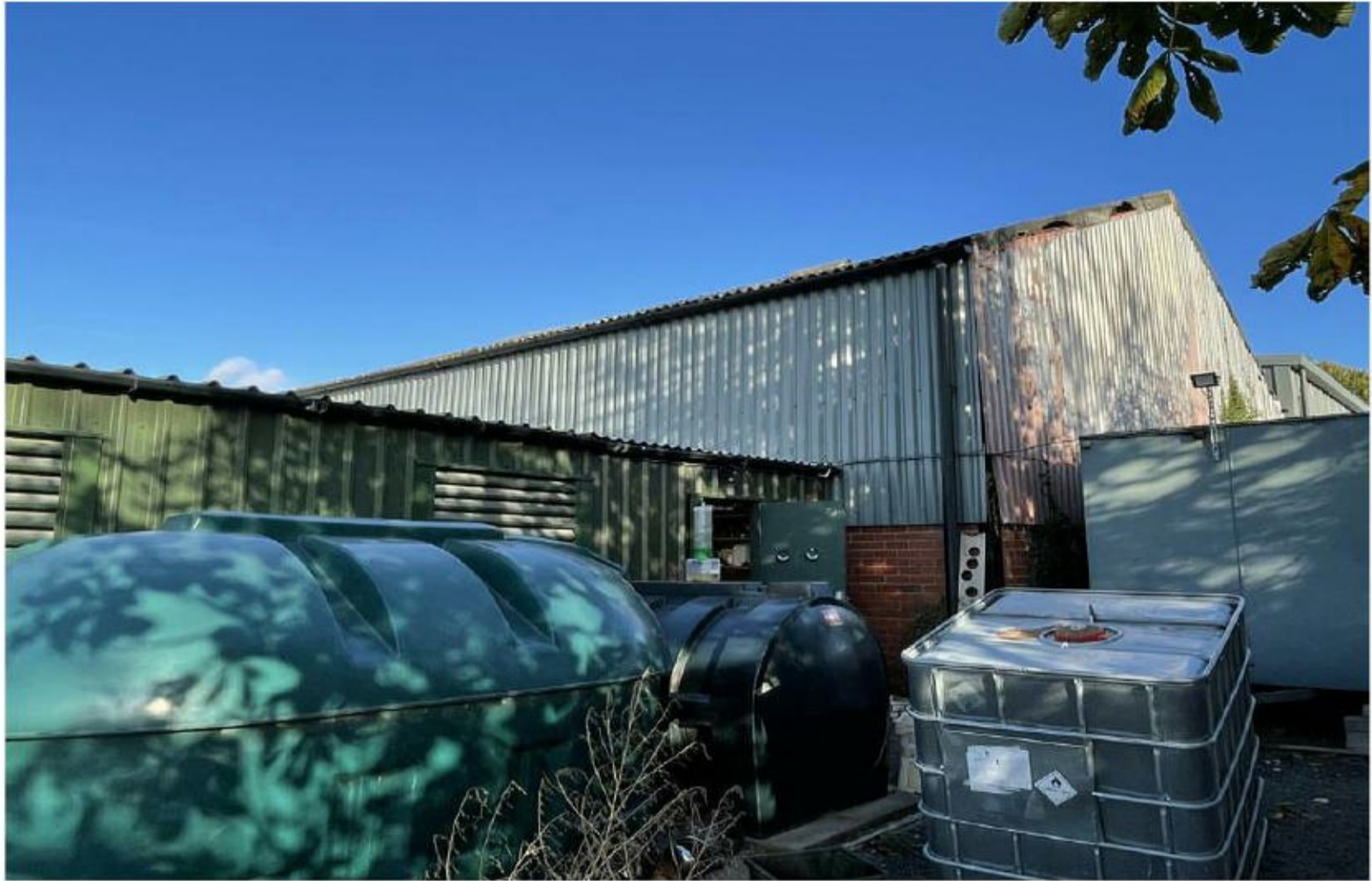
Photograph 8: Southern elevation of Billy's Barn and attached building
