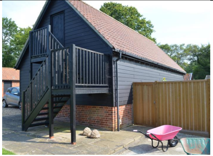
Photo 2 Cart lodge where an extension is proposed
