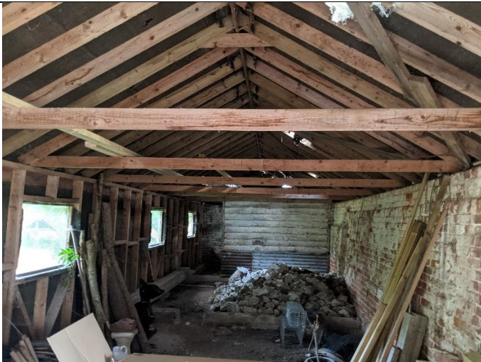
Photo 3 Internal view of the outbuilding
