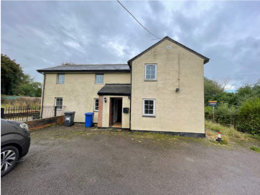
North (side) elevation as seen from driveway
