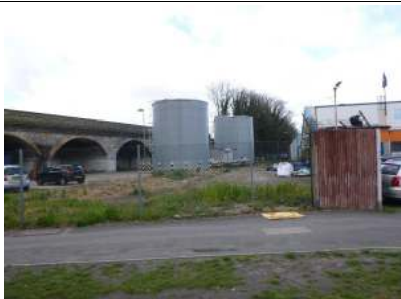
View to the west showing the two large tanks understood to contain water which feeds the fire sprinkler system of the retail units located to the west of the site.
