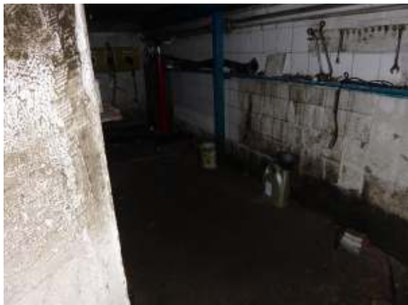
Vehicle inspection pit at western end of workshop.
