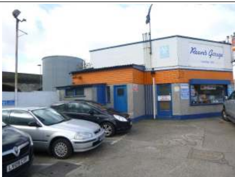
Looking west towards existing garage building from eastern edge of the site.
