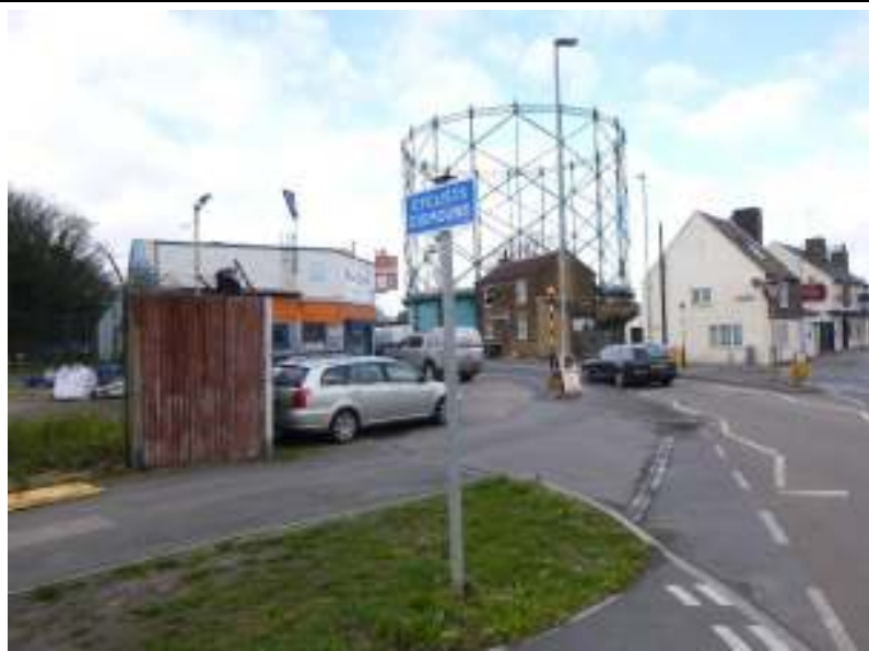
View to the northwest looking across the south. The gas holder present to the north west of the site can be seen in the background.
