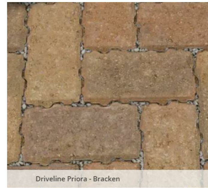
PERMEABLE PAVING FOR FOOT PATHS, WALK WAYS AND PARKING SPACES. TO BE INSTALLED ACCORDING TO MANUFACTURE'S DETAILS (PLEASE SEE DEAILING FOR MORE INFORMATION ON BUILD UP
