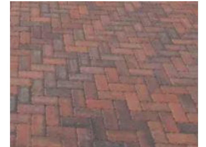
PERMEABLE PAVING FOR DRIVE WAYS AND WALK WAYS. TO BE INSTALLED ACCORDING TO MANUFACTURE'S DETAILS (PLEASE SEE DEAILING FOR MORE INFORMATION ON BUILD UP
