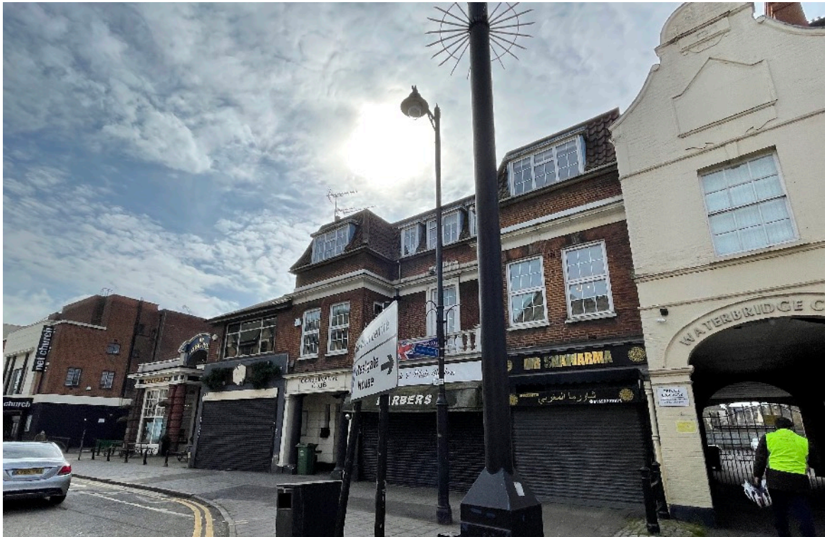
Fig. 3 - 48 Spital Street, Neighbouring Property
