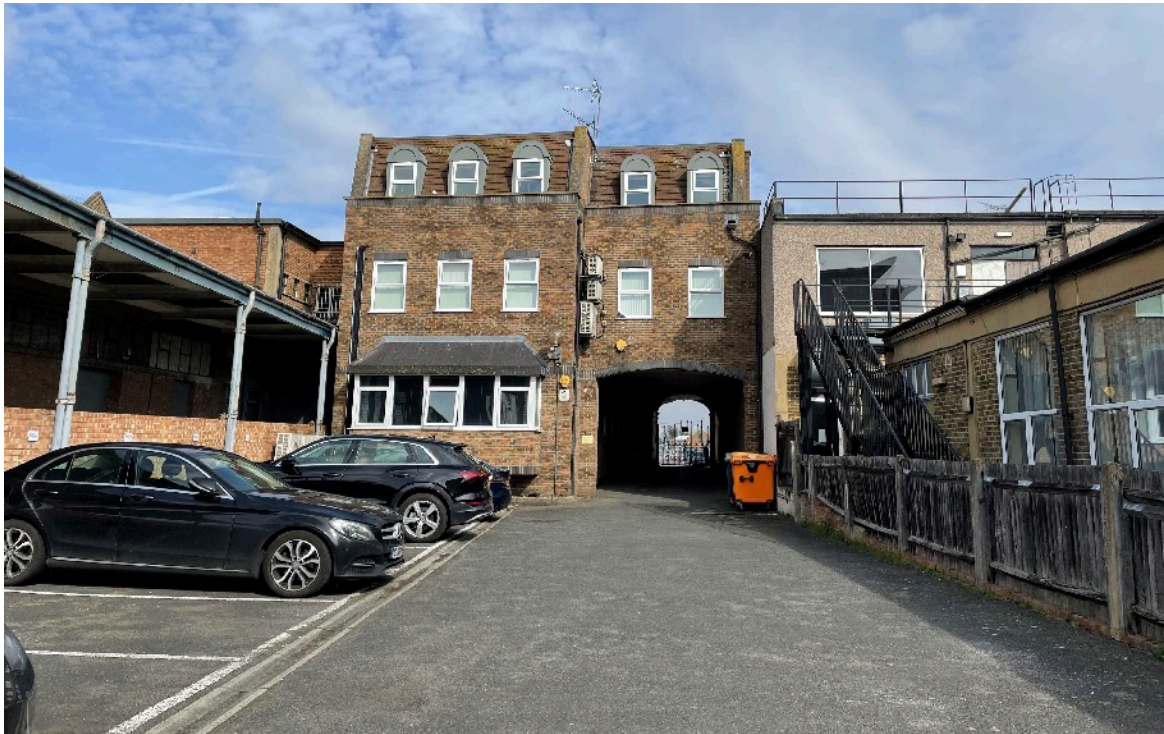
Fig. 5 - Rear Elevation from car park
