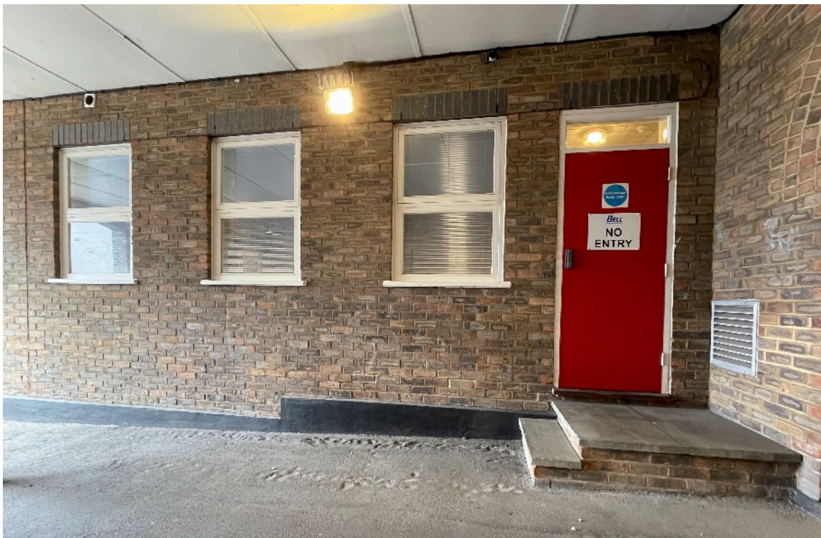
Fig. 4 - Ground Floor Side Entrance
