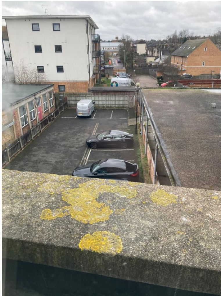
Fig. 8 - Existing rear Car Parking
