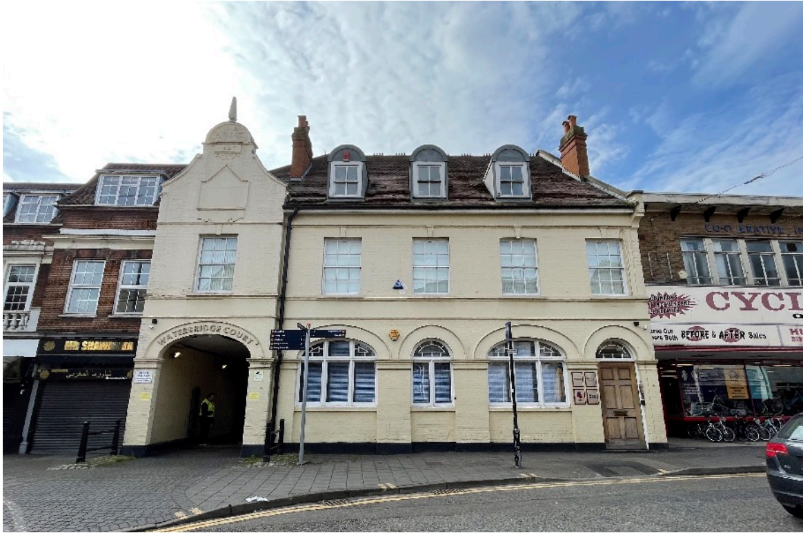
Fig. 1 - Front Facade, 50 Spital Street
