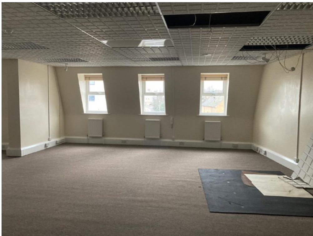
Fig. 9 - Internal condition of Second Floor
