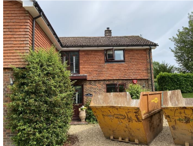
View of Northwest elevation from driveway.
