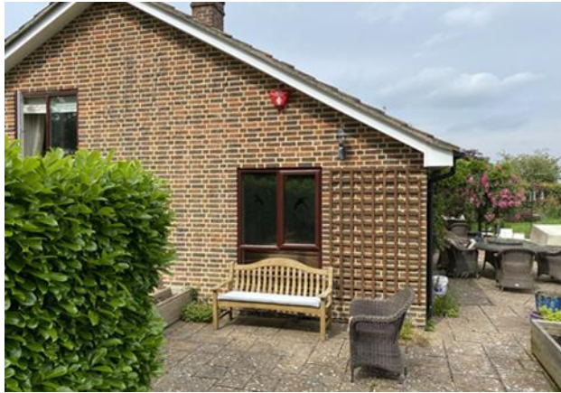
View of Southwest elevation towards the rear patio.
