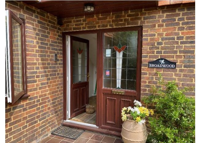
View of existing porch entrance.
