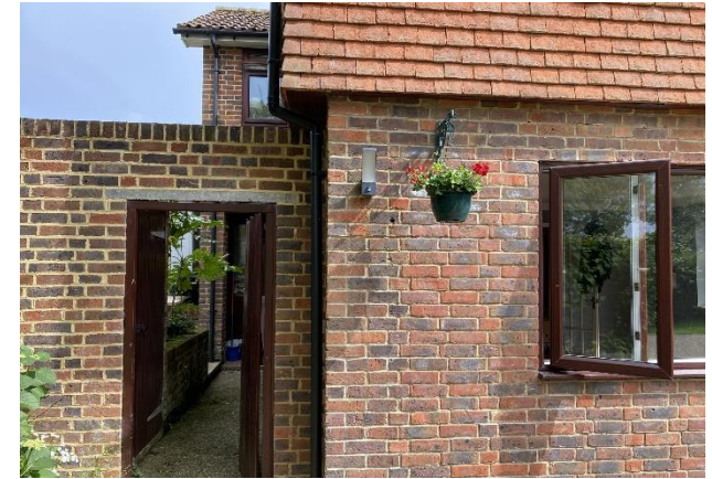
View of side entrance of Northwest elevation.
