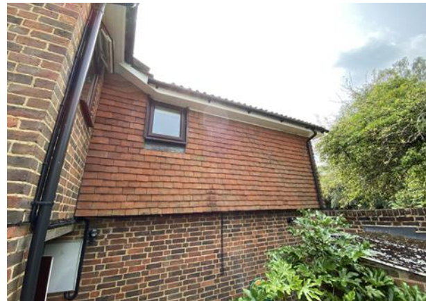
View of Northeast elevation.
