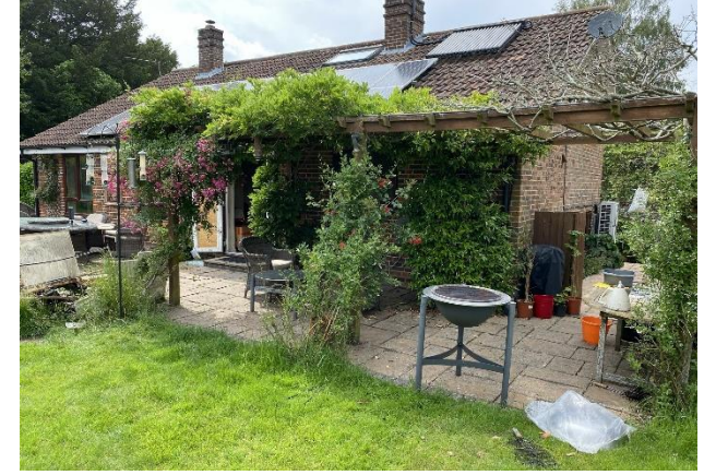
View of the existing pergola to be removed.
