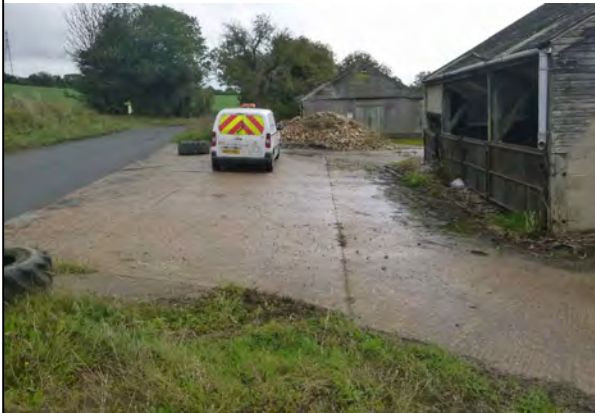
Photo 2 - Compacted gravel/hard-core along the western boundary
