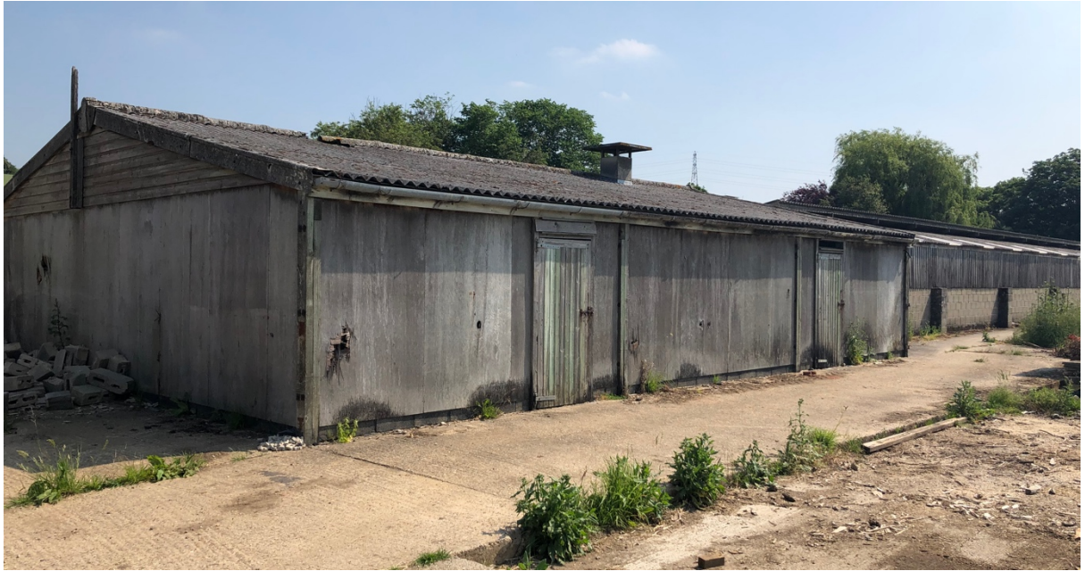
Picture 5 – Barn C (foreground), to be converted to 1no. dwelling
