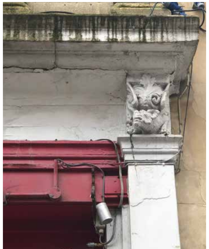
Close up - Original detailing on front facade
