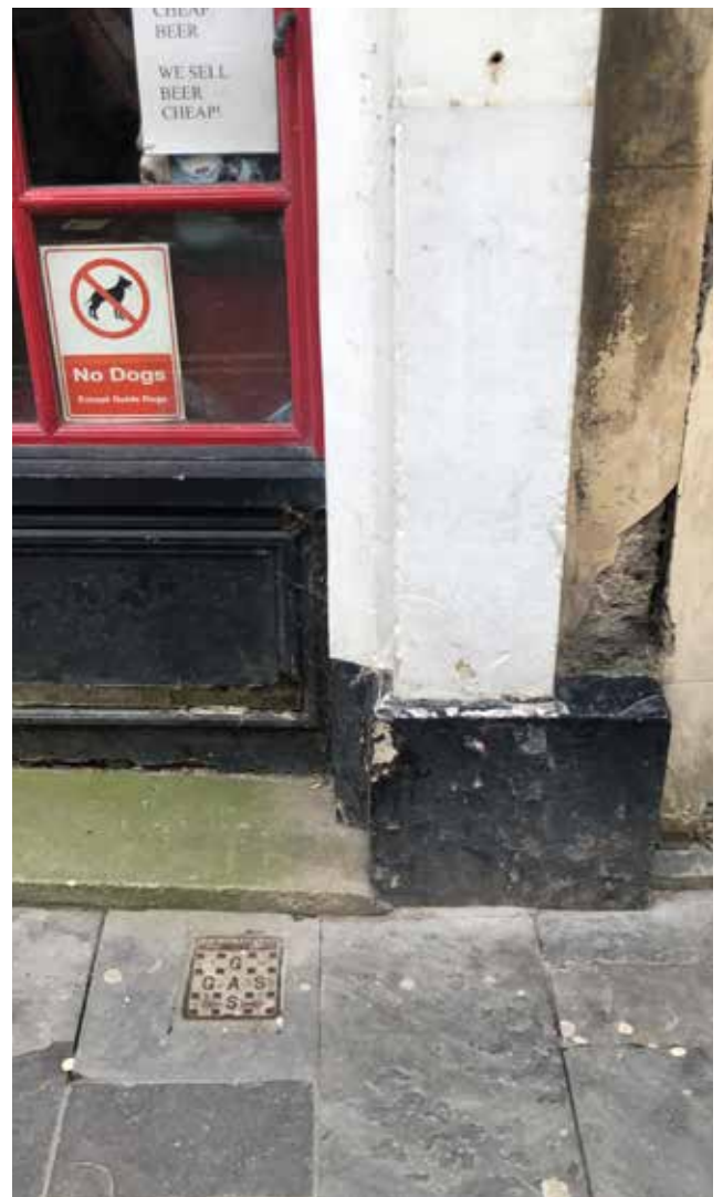
Connection between No 132 shopfront and existing Pilaster
