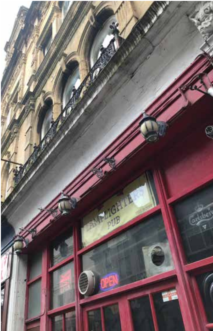
Lamp lighters existing shopfront and pre-existing details
