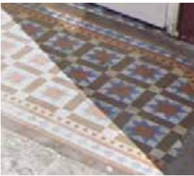
Existing tiles to entrances
