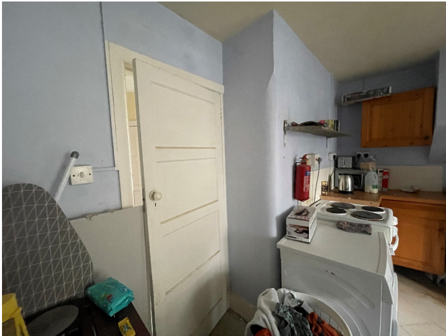
Point No 2. Existing kitchen doorway kept and create small new w/c
