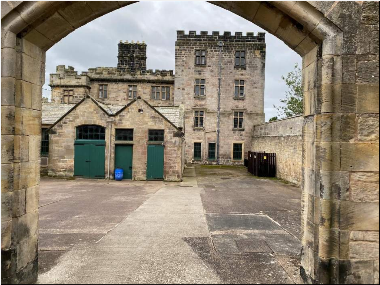
Plate 5: Ford Castle eastern front (1371004) with service wing to foreground (1042186)
