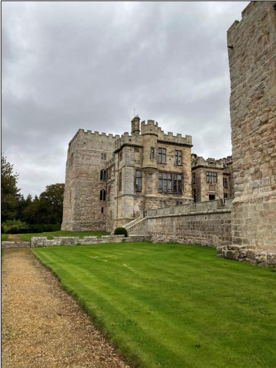
Plate 3: Ford Castle western end of southern (entrance) front (1371004) including King James Tower to LHS
