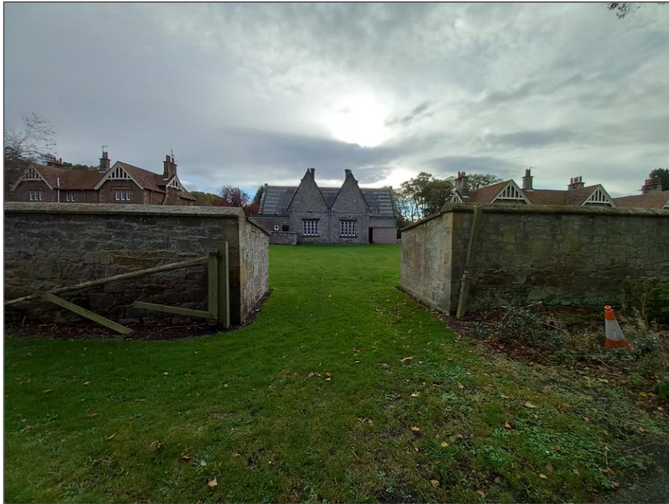
Plate 15: Rear of Lady Waterford Hall (1042153)
