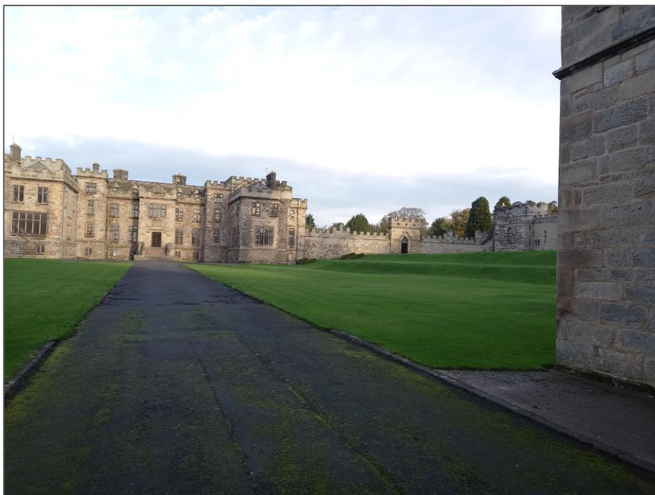
Plate 2: Oblique view of Ford Castle (1371004) from the southern gateway. Site not visible
