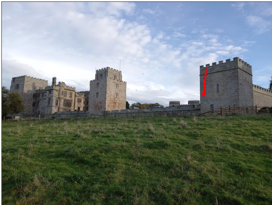
Plate 4: View of Ford Castle (1371004) from the south-west. Site not visible – tallest element (zip wire) would be to the rear of built form
