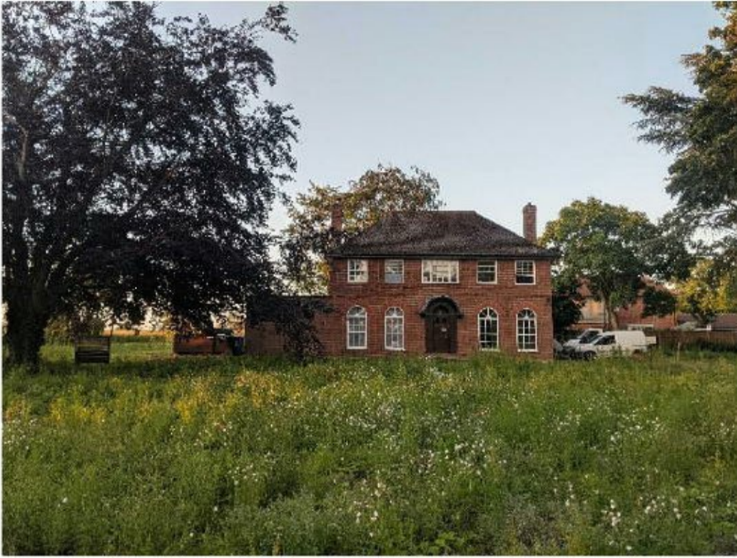
Photo 1 Southwest elevation of Rathkeltair Lodge
