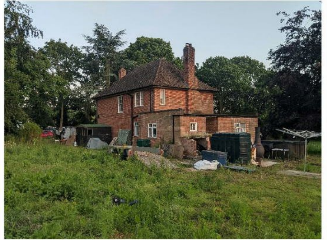
Photo 2 Northwest and northeast elevations of dwelling
