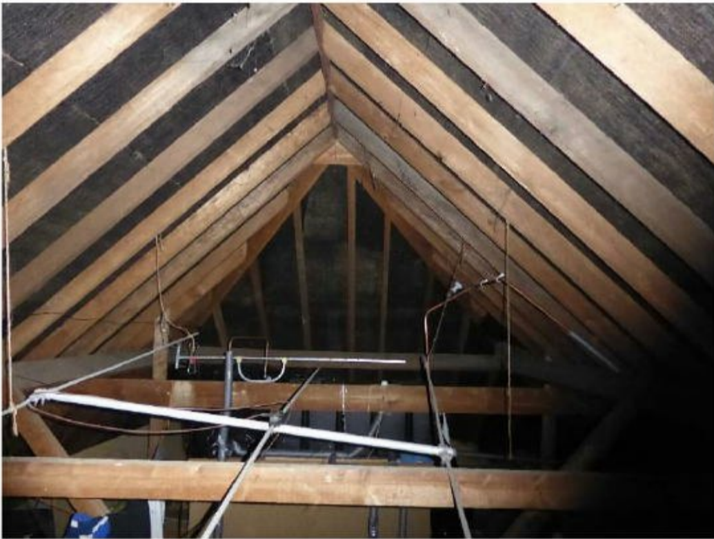
Photo 9 Roof void of Rathkeltair Lodge
