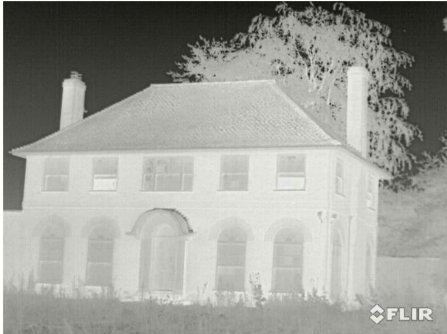
Plate 1 West and south elevations of Rathkeltair Lodge – 14/07/21
