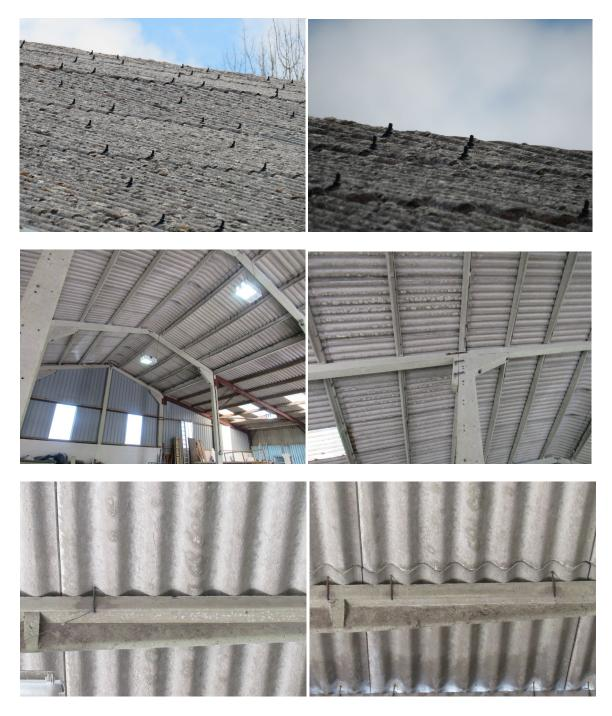
There is a gap between the rear of the fibre cement roof sheets and the concrete sheeting rail but the likelihood of this being used by bats is exceptionally small and highly unlikely.
