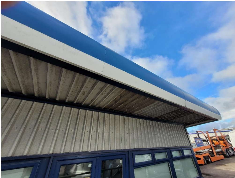
Plate 8 – former sales office - western elevation
