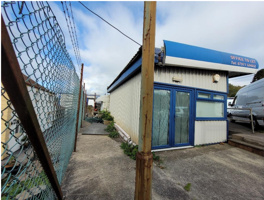
Plate 7 – former sales office - southern and western elevations
