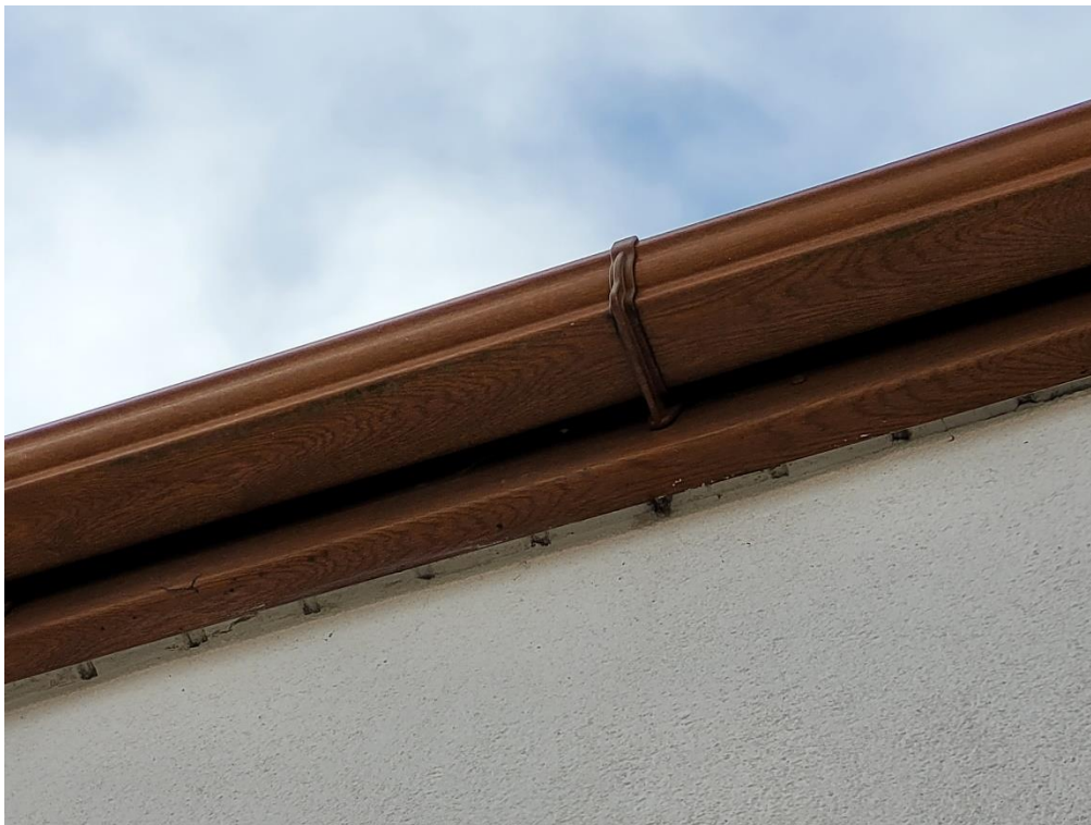
Plate 5a – uPVC fascia / soffit detail
