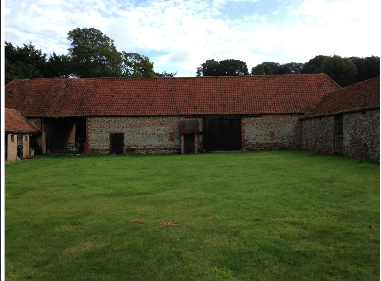
Above -Photos showing position and condition of red diesel tank (not in use at time of photos 2017).
