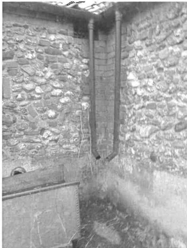
P5: Southern single storey barn: Poor roof detailing to valley of courtyard facing return
