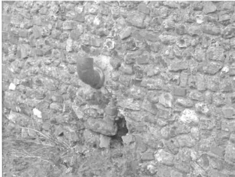
P1: Southern single storey barn: Small void at low level to courtyard facing north elevation
