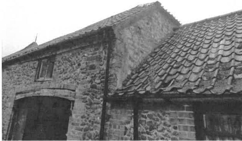
P11: West Wing: Significant diagonal cracking above main arched opening into two storey barn section
