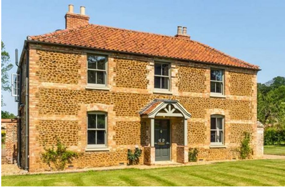
Image 2: Example of external joinery colour used across the wider estate
