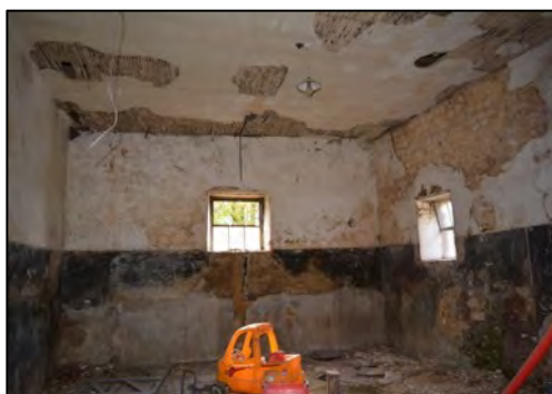
Figure 28 – Internal view of Main Barn 4 Complex (Section I) showing the lath and plaster ceiling including gaps
