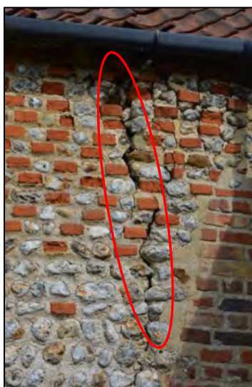
Figure 30 – External feature on the western elevation of Main Barn 4 Complex (section C)
