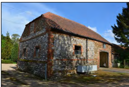
Figure 20 – North-western view of Barn 4 Complex (section I)
