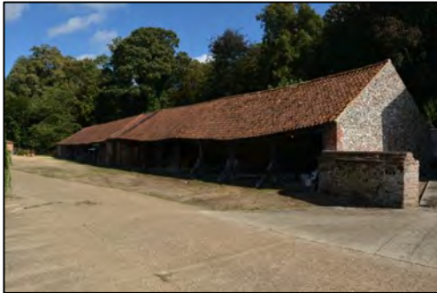
Figure 11 – Eastern view of Field Barn 3
