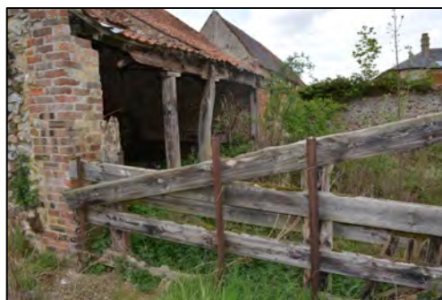
Figure 21 – Eastern view of Main Barn 4 Complex (section G), showing the overgrown area to the east of the barn
