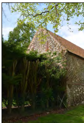
Figure 9 – Southern elevation of Field barn 2
