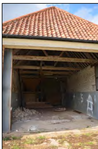
Figure 22 – Southern view of Main Barn 4 Complex (section C), Barn Owl pellets were noted towards the entrance of the barn
