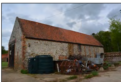
Figure 5 – Southern elevation of Field Barn 1
