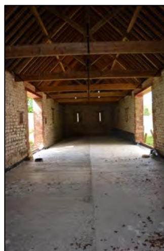
Figure 8 – Internal view of Field Barn 2 looking north
