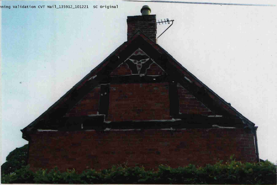
PHOTOGRAPH 3 - DETAIL OF THE EXPOSED TIMBER FRAMING WITH THE END GABLE.
