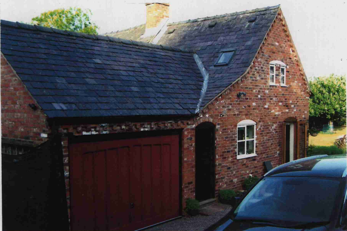
PHOTOGRAPH 4 - GENERAL VIEW OF THE LATE 1990'S EXTENSION AT THE OTHER END OF THE HOUSE.
