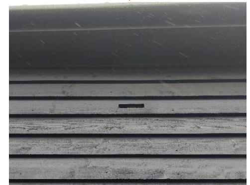
Access to the bat boxes cut into the weather boarding. The holes can be cut by scalloping the underside of the board where it covered the board below to reduce water ingress
