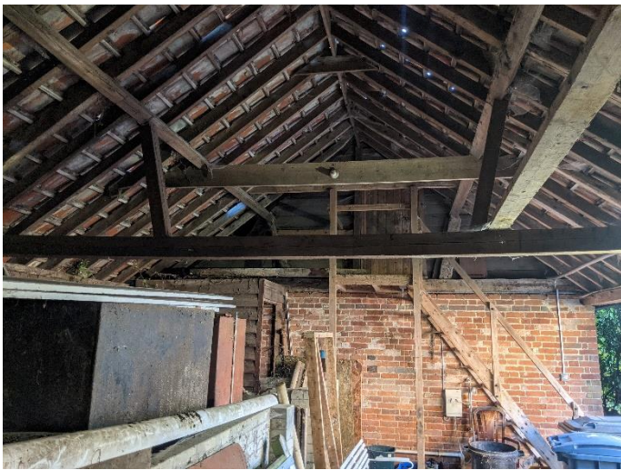
Photo 9 Internal view of the cart shed
