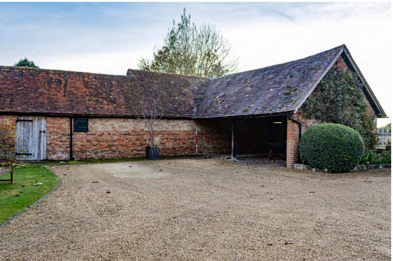
Plate 8 (001): Cow Shed, South-West Elevation, general view from the west
