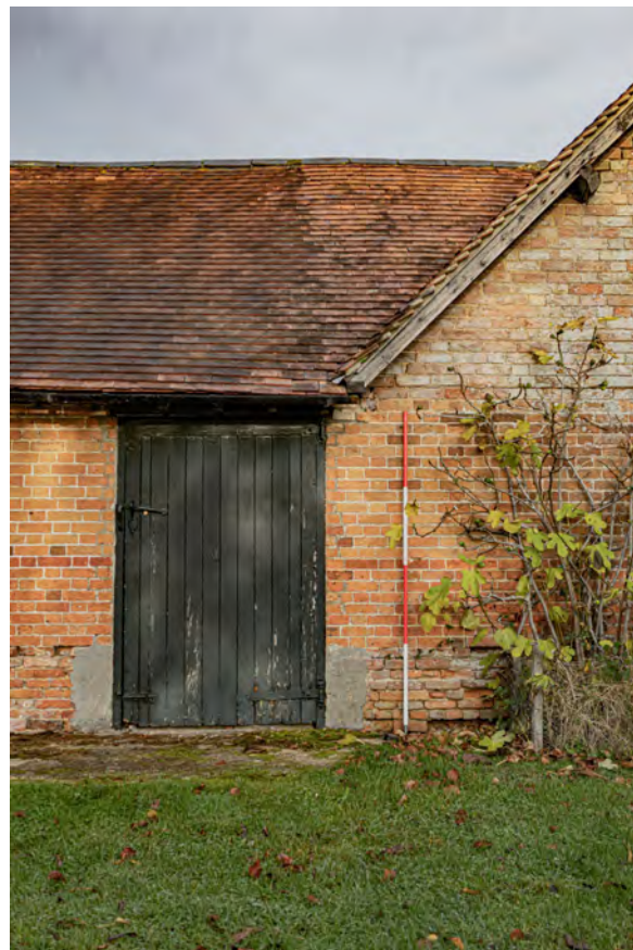
Plate 40 (031): Cart Store, South-East Elevation, detail of doorway [15] from the south-east
