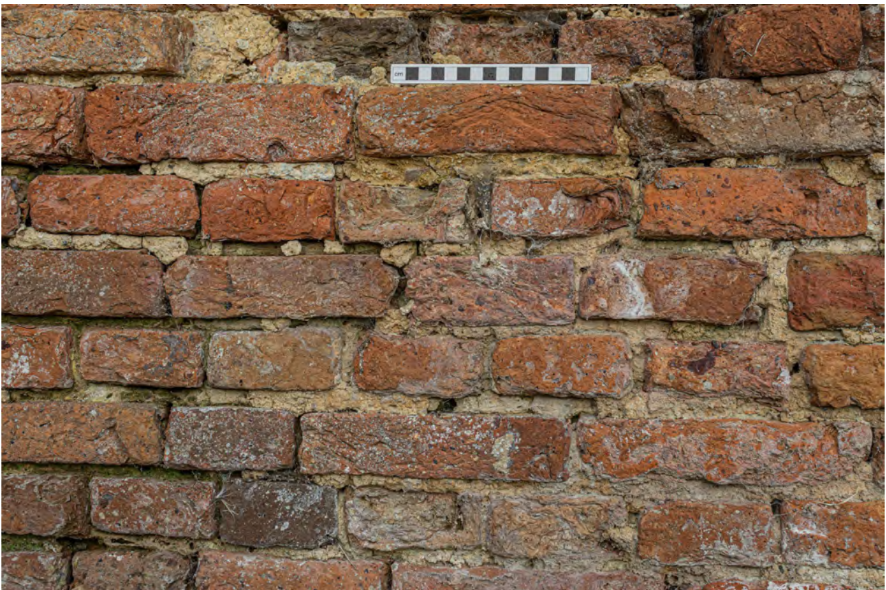
Plate 38 (032): Cart Store, South-East Elevation, detail of brick wall [13] from the south-east
