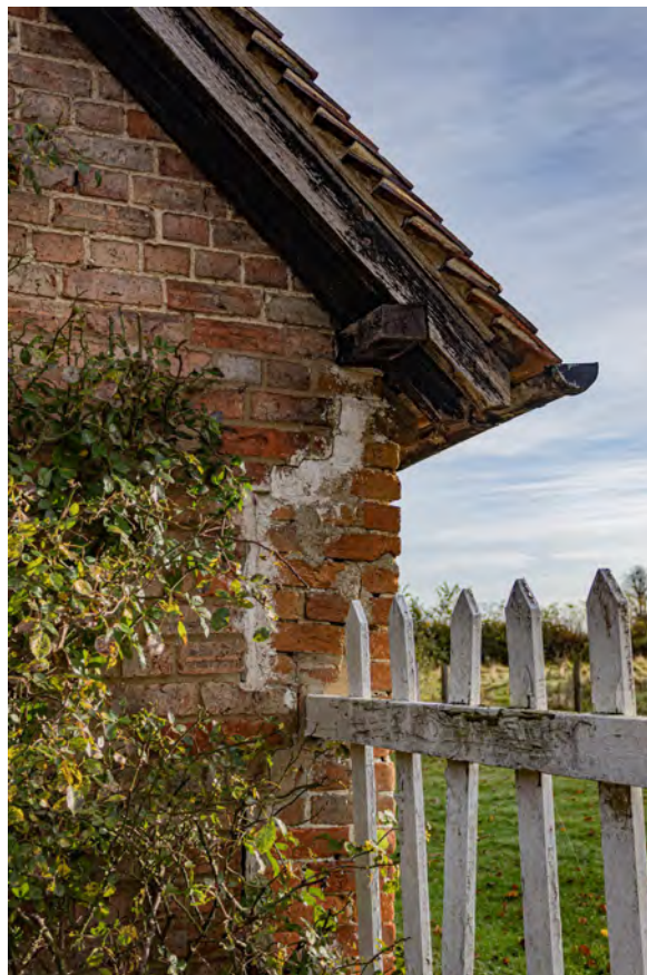
Plate 34 (026): Cart Store, South-West Elevation, detail of the scar for the former rainwater goods, from the south-west
