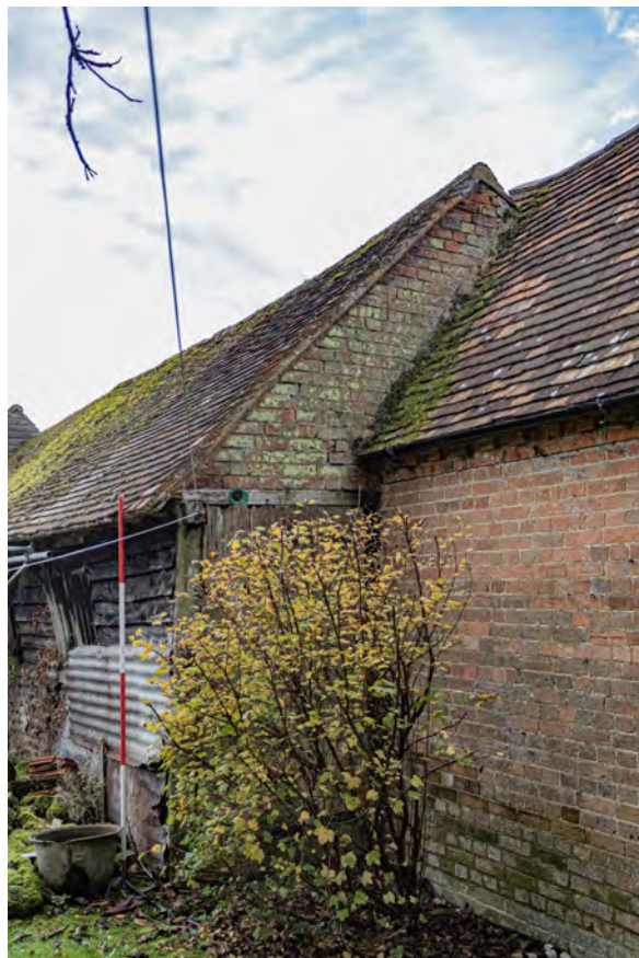
Plate 58 (049): Cow Shed, North-West Elevation, general view from the north
