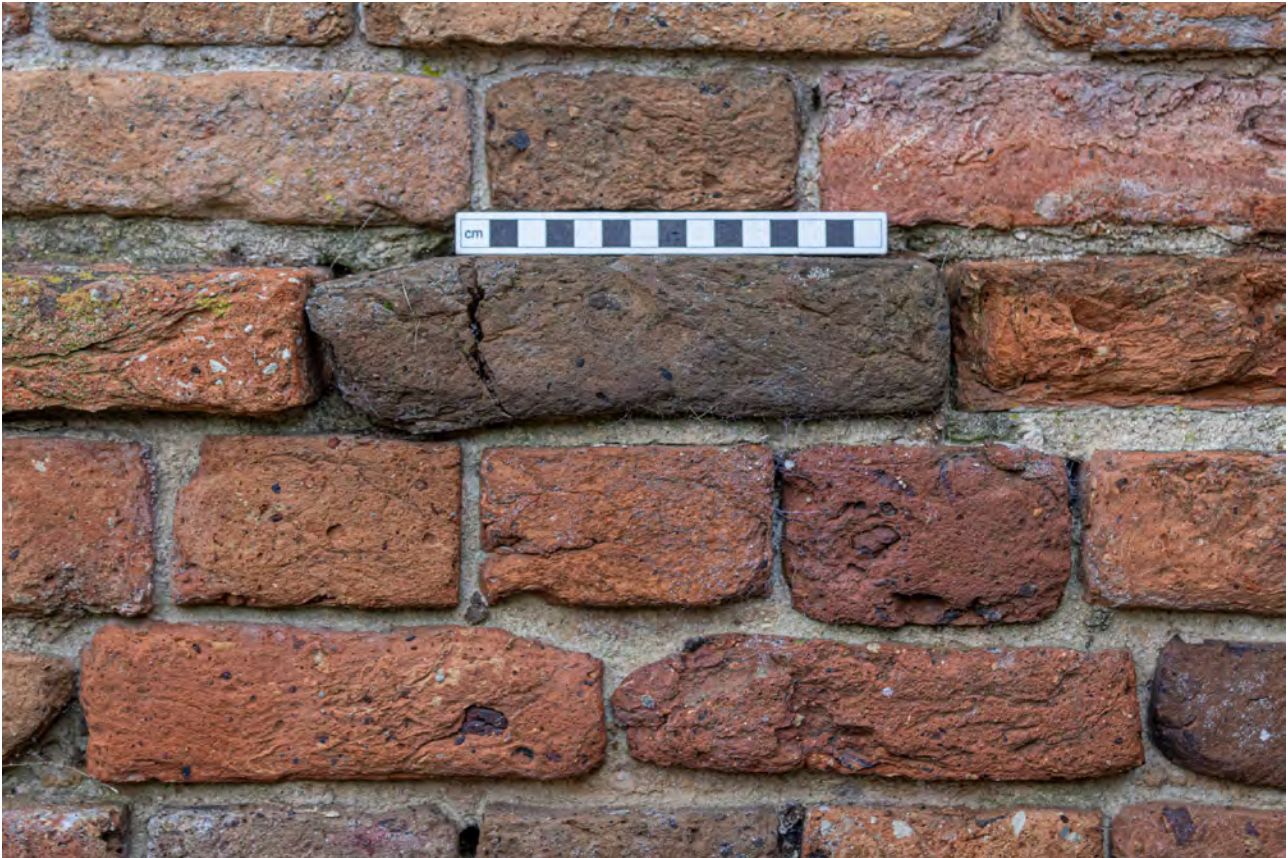
Plate 13 (018): Cow Shed, South-West Elevation, detail of wall [01] from the south-west
