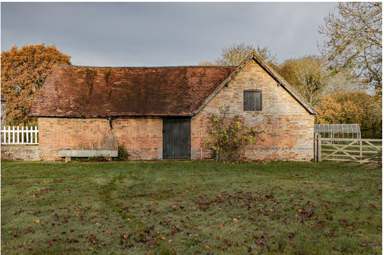
Plate 36 (027): Cart Store, South-East Elevation, general view from the south-east
