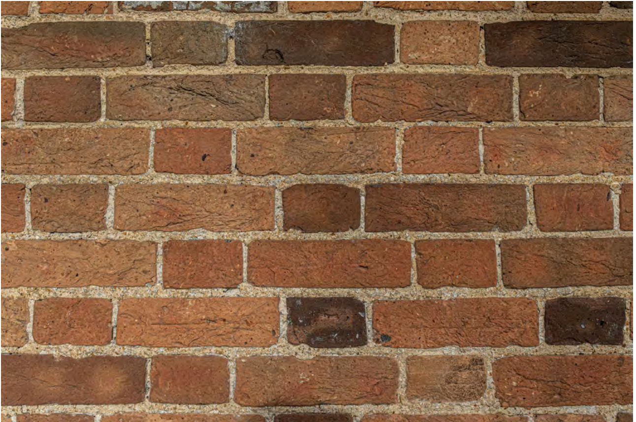
Plate 39 (033): Cart Store, South-East Elevation, detail of brick wall [14] from the south-east
