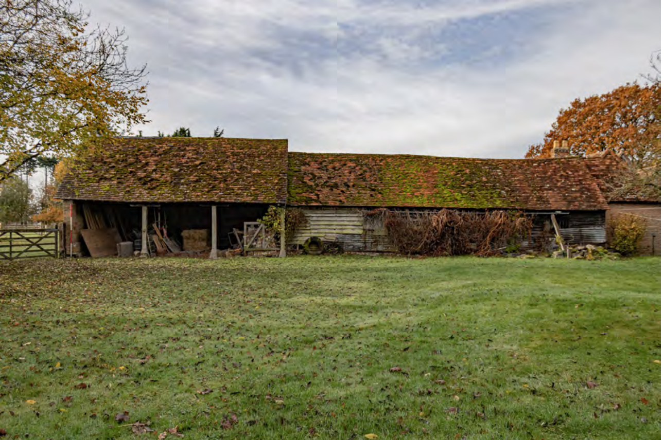
Plate 45 (035): Cart Store, North-East Elevation, general view from the north-east
