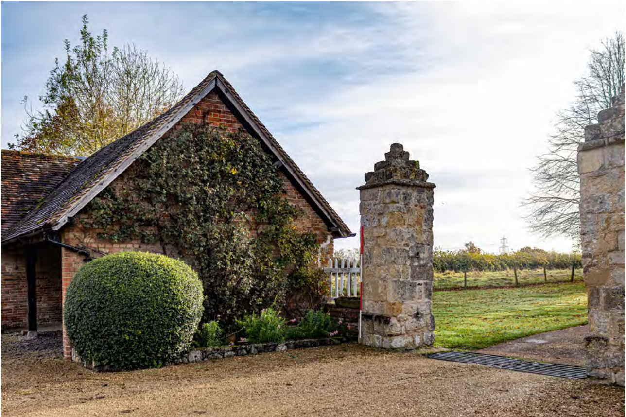
Plate 31 (023): Cart Store, South-West Elevation, general view from the west
