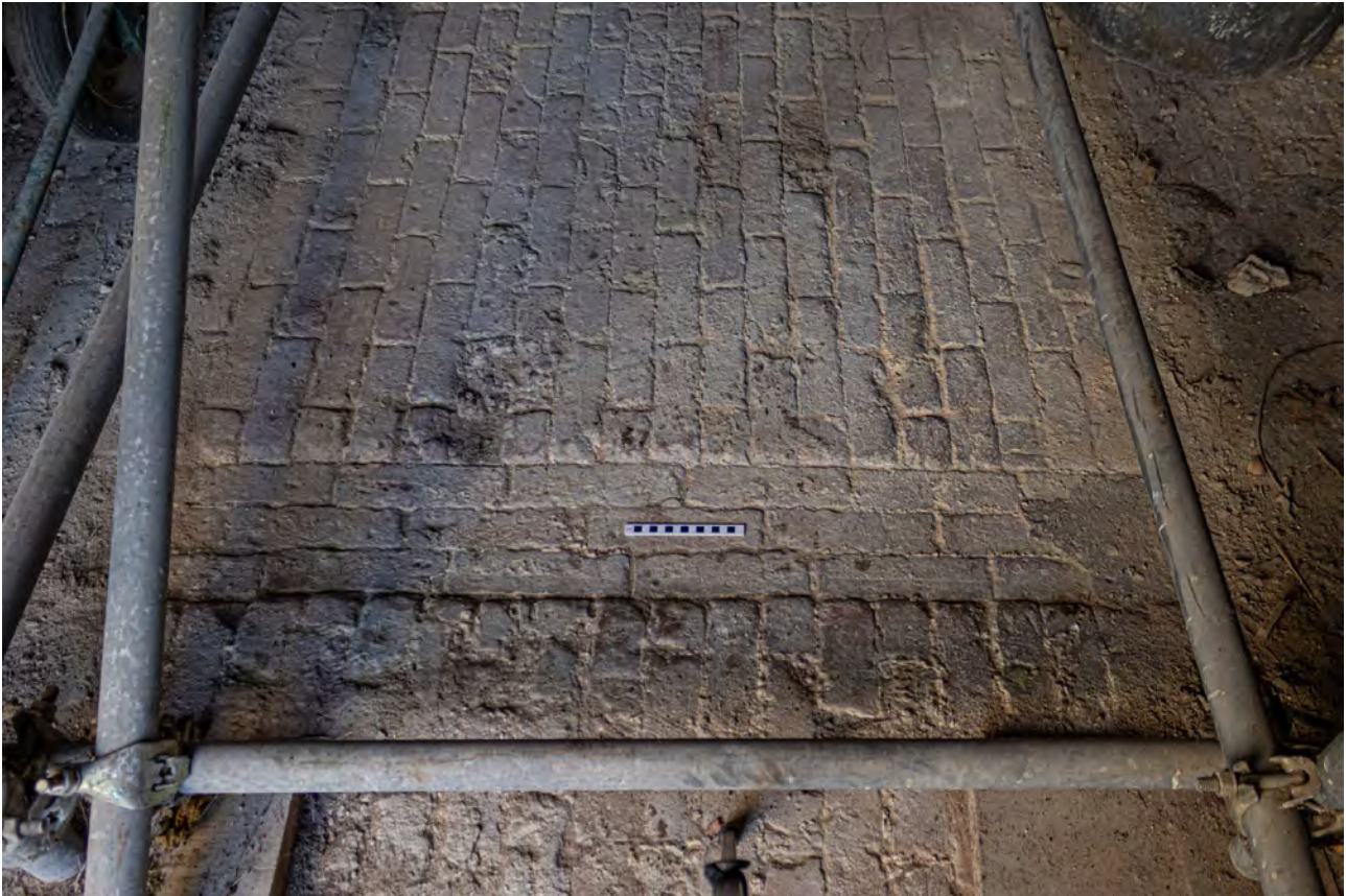
Plate 71 (060): Room 1, detail of brick floor and drain from the south-west
