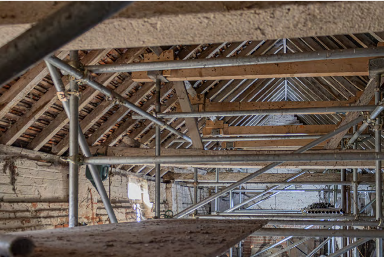
Plate 65 (071): Room 1, general view from the SSE
