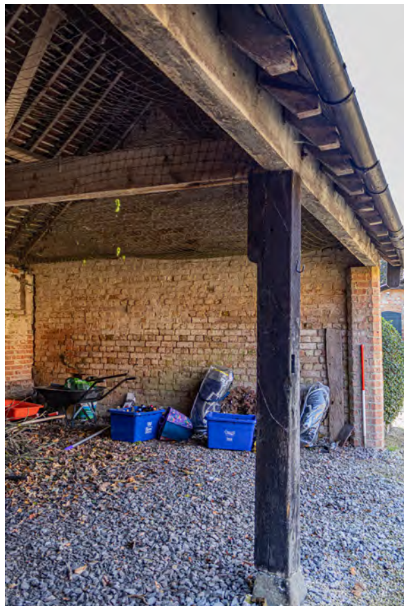
Plate 26 (077): Cart Store, North-West Elevation, detail of post from the ENE
