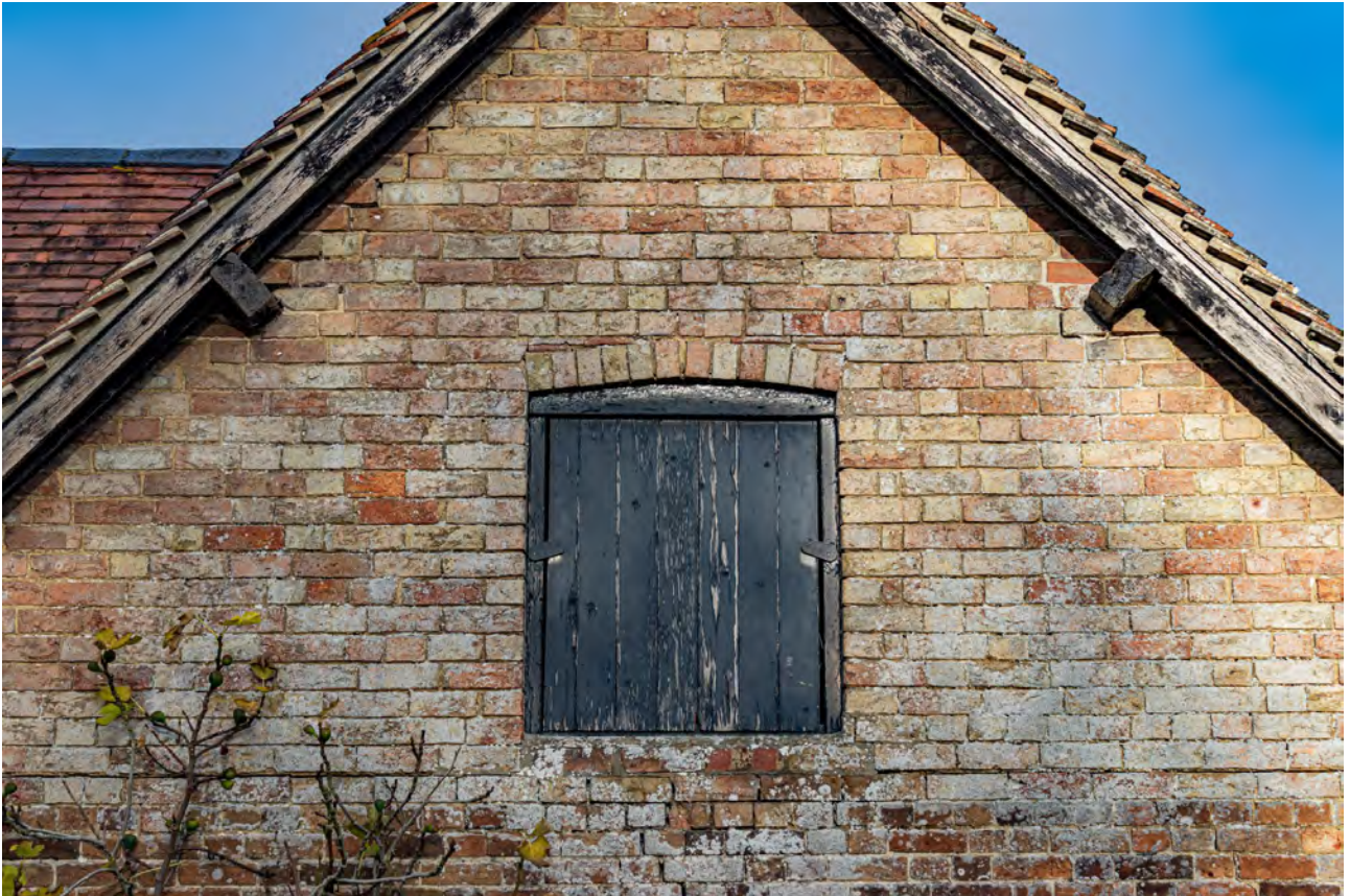
Plate 43 (030): Cart Store, South-East Elevation, detail of attic hatch from the south-east
