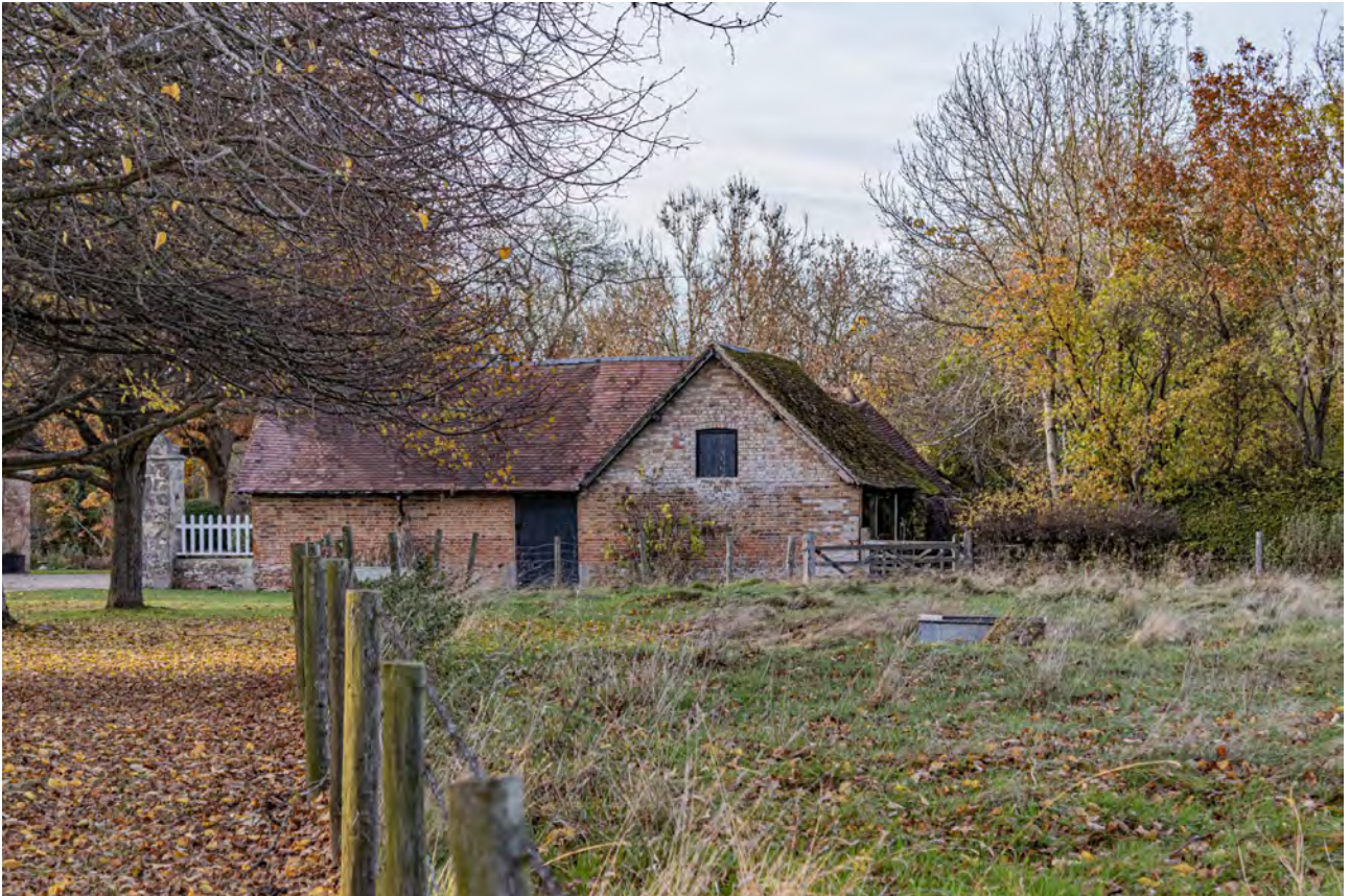
Plate 35 (119): Cart Store, South-East Elevation, general view from the SSE
