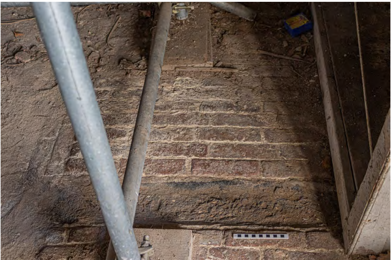
Plate 72 (064): Room 1, detail of brick floor and drain from the north-west
