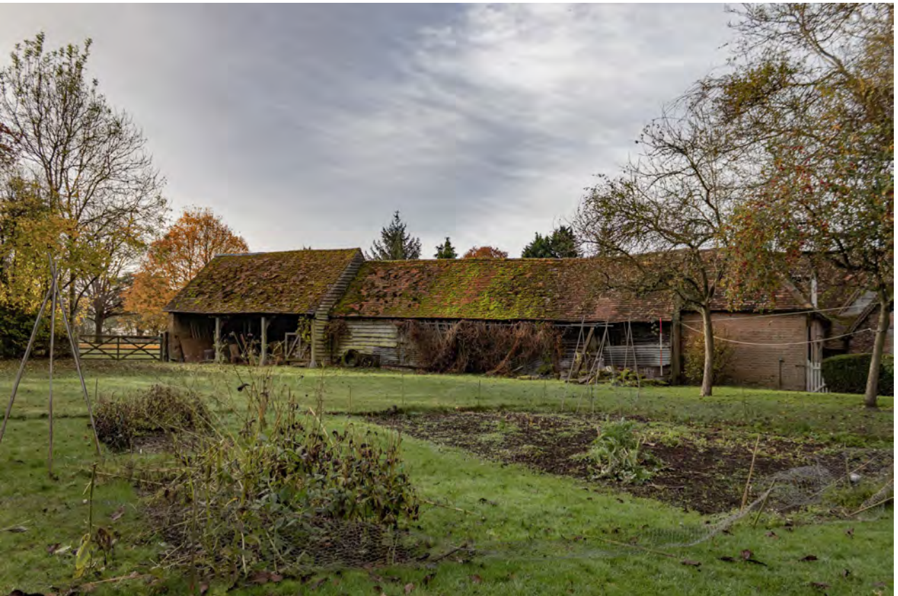
Plate 46 (039): Cart Store, North-East Elevation, general view from the NNE
