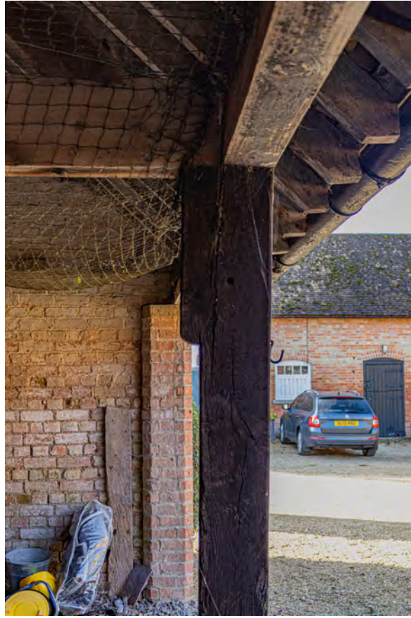
Plate 27 (081): Cart Store, North-West Elevation, detail of post from the north-west
