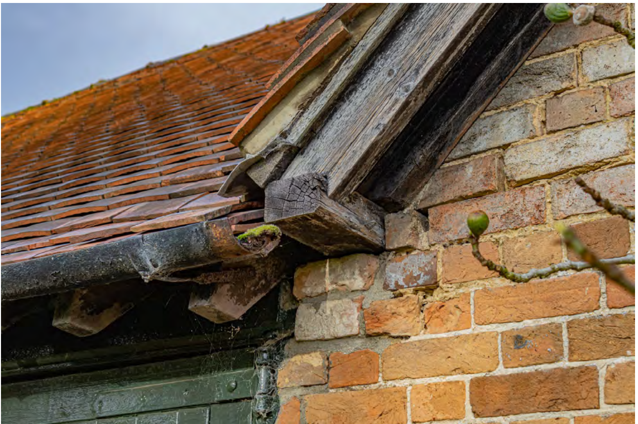
Plate 42 (034): Cart Store, South-East Elevation, detail of beam in the east
