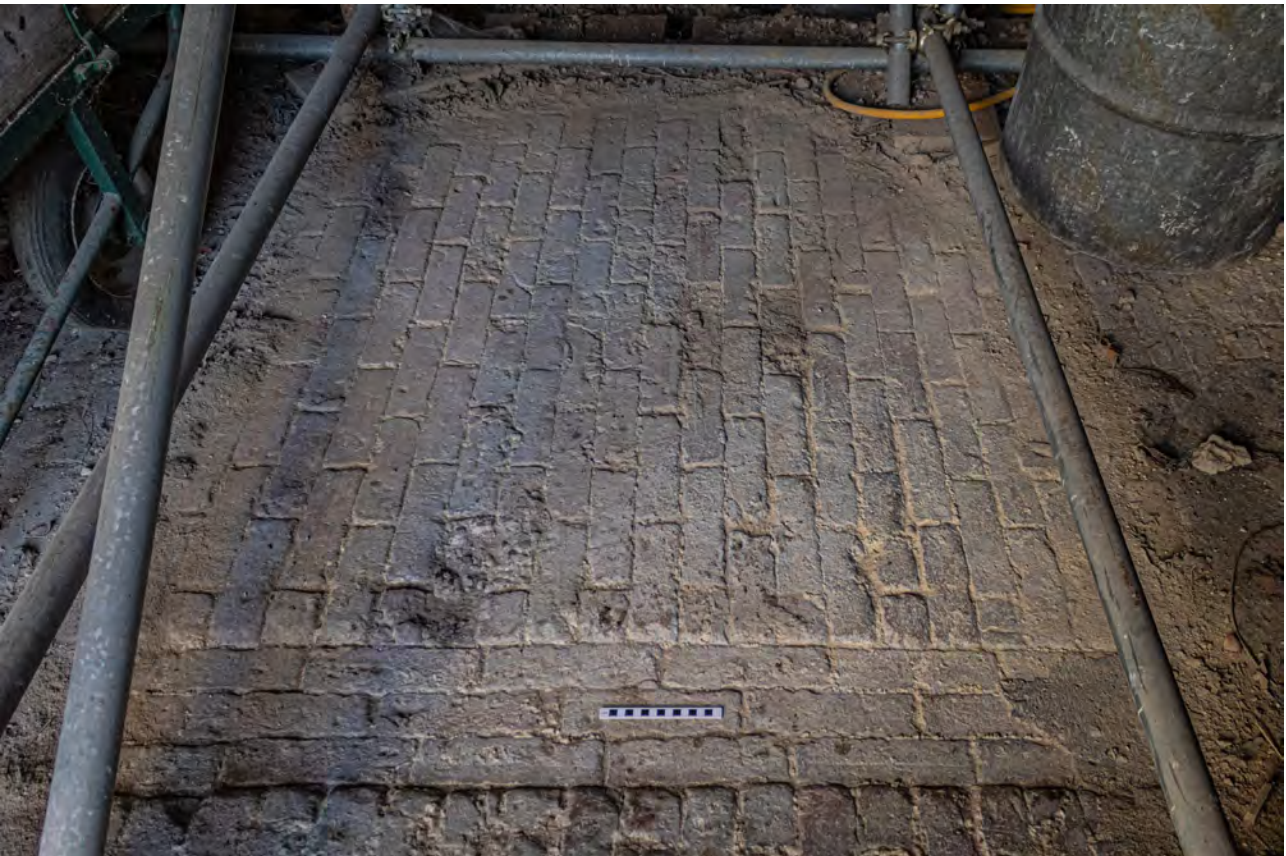
Plate 70 (061): Room 1, detail of brick floor and drain from the south-west
