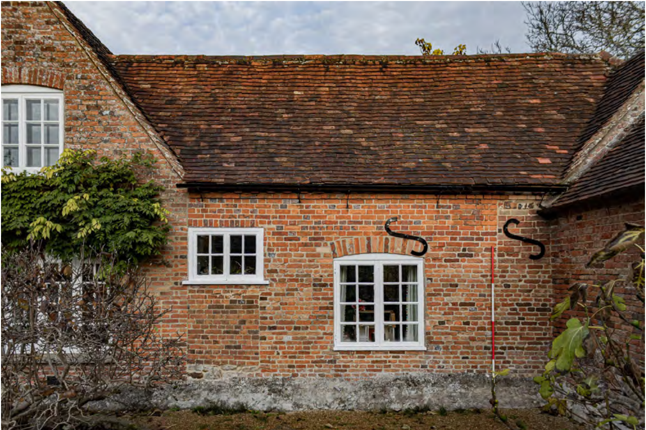
Plate 61 (012): Farmhouse, South-East Elevation, general view from the south-east
