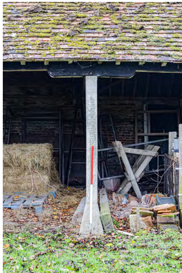
Plate 50 (040): Cart Store, North-East Elevation, detail of post [19] from the north-east
