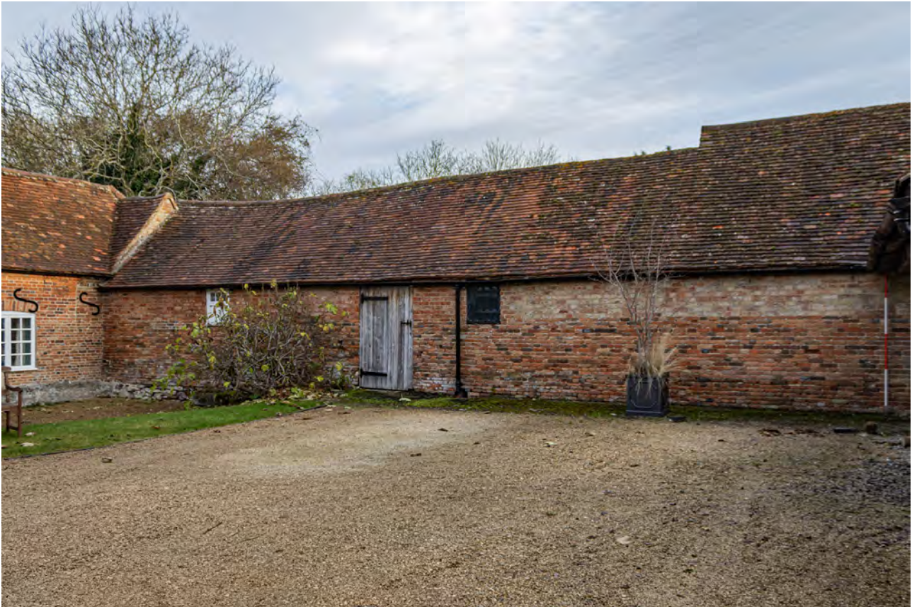
Plate 11 (004): Cow Shed, South-West Elevation, general view from the WSW
