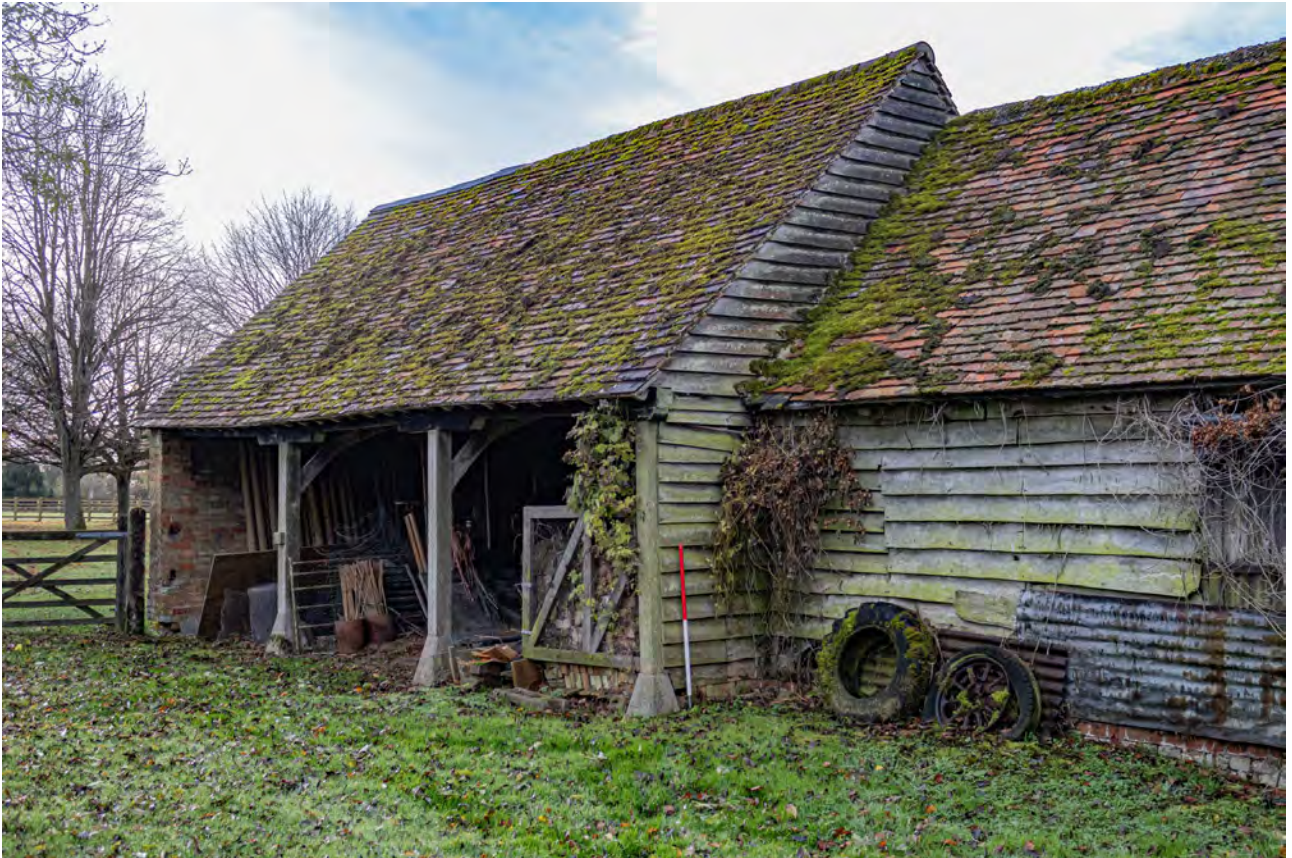
Plate 49 (044): Cart Store, North-East Elevation, general view from the west
