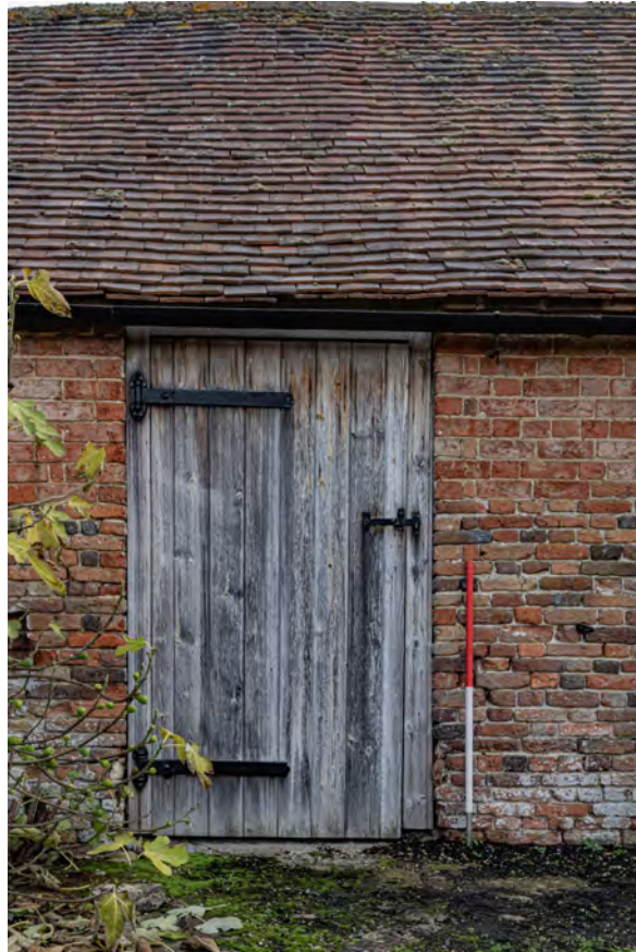
Plate 17 (006): Cow Shed, South-West Elevation, detail of doorway [04] from the south-west
