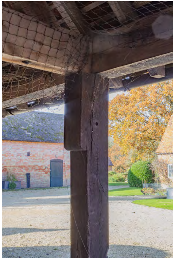
Plate 28 (082): Cart Store, North-West Elevation, detail of post from the south-east
