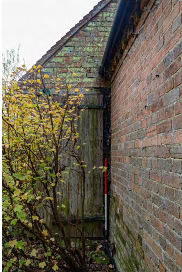
Plate 59 (052): Cow Shed, North-West Elevation, detail of door [25] from the north-west
