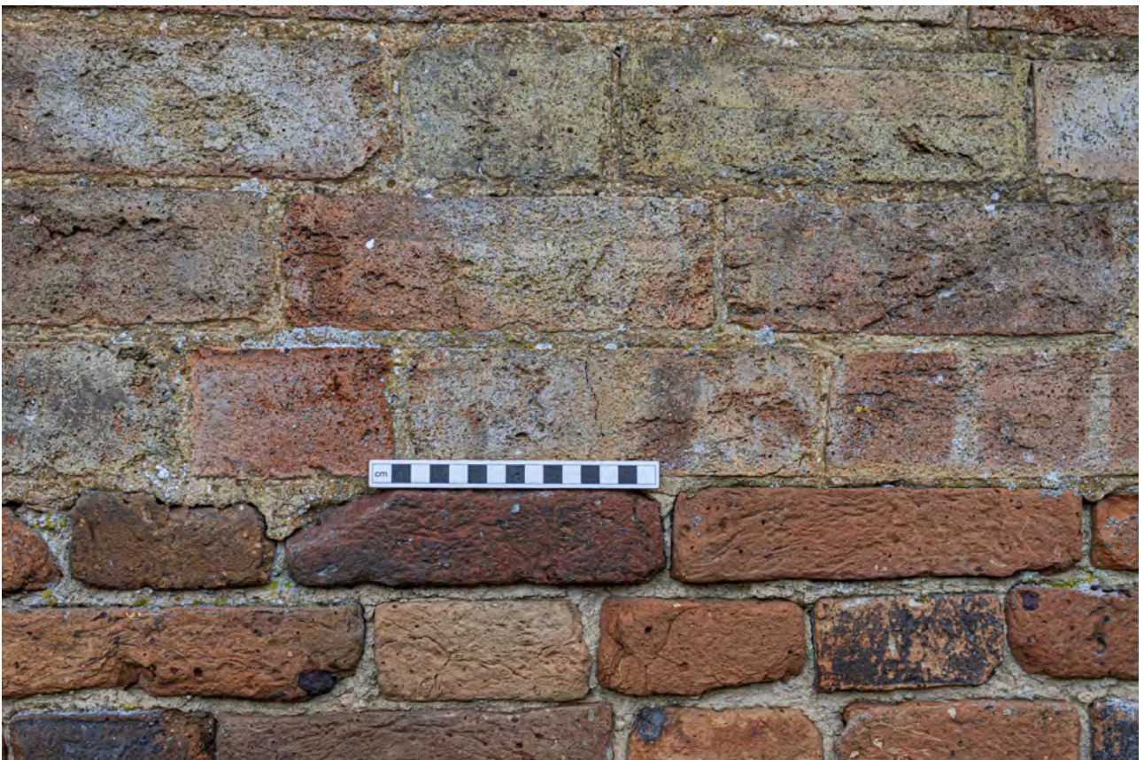
Plate 16 (015): Cow Shed, South-West Elevation, detail of wall [03] from the south-west
