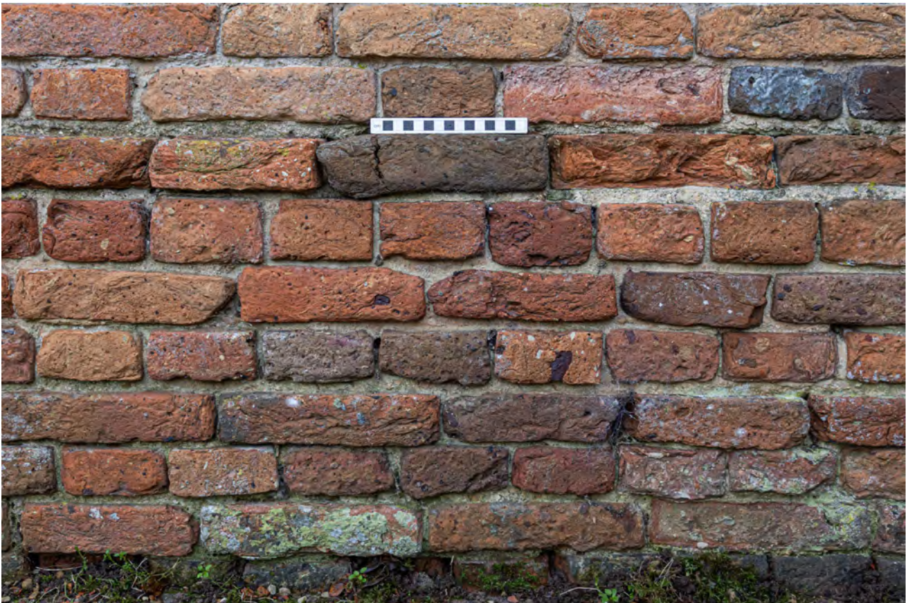
Plate 12 (017): Cow Shed, South-West Elevation, detail of wall [01] from the south-west
