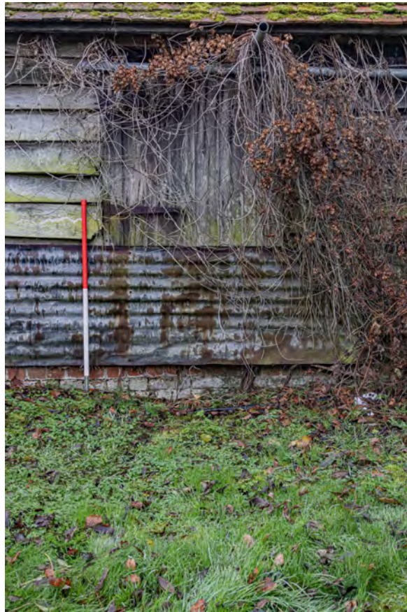
Plate 53 (046): Cow Shed, North-East Elevation, detail of south-easternmost hatch from the north-east
