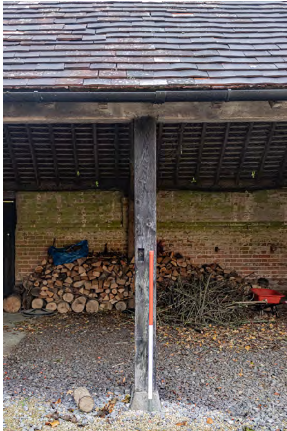
Plate 25 (021): Cart Store, North-West Elevation, detail of post from the north-west
