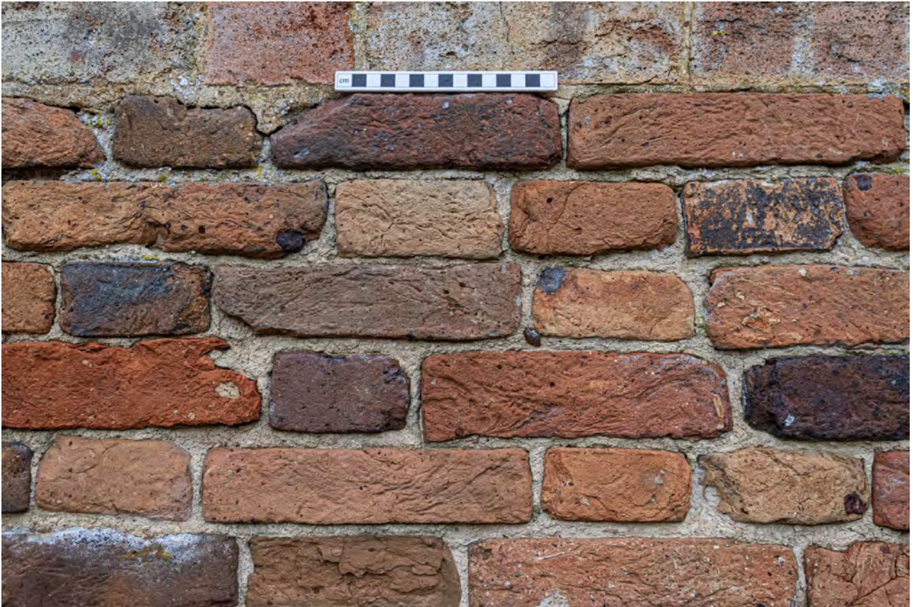
Plate 15 (016): Cow Shed, South-West Elevation, detail of wall [02] from the south-west
