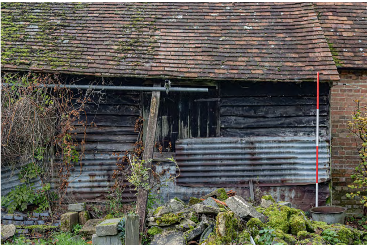
Plate 54 (047): Cow Shed, North-East Elevation, detail of north-westernmost hatch from the north-east
