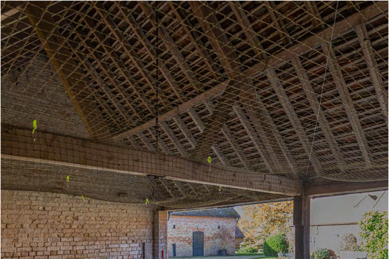
Plate 123 (079): Room 3, detail of Truss G from the east
