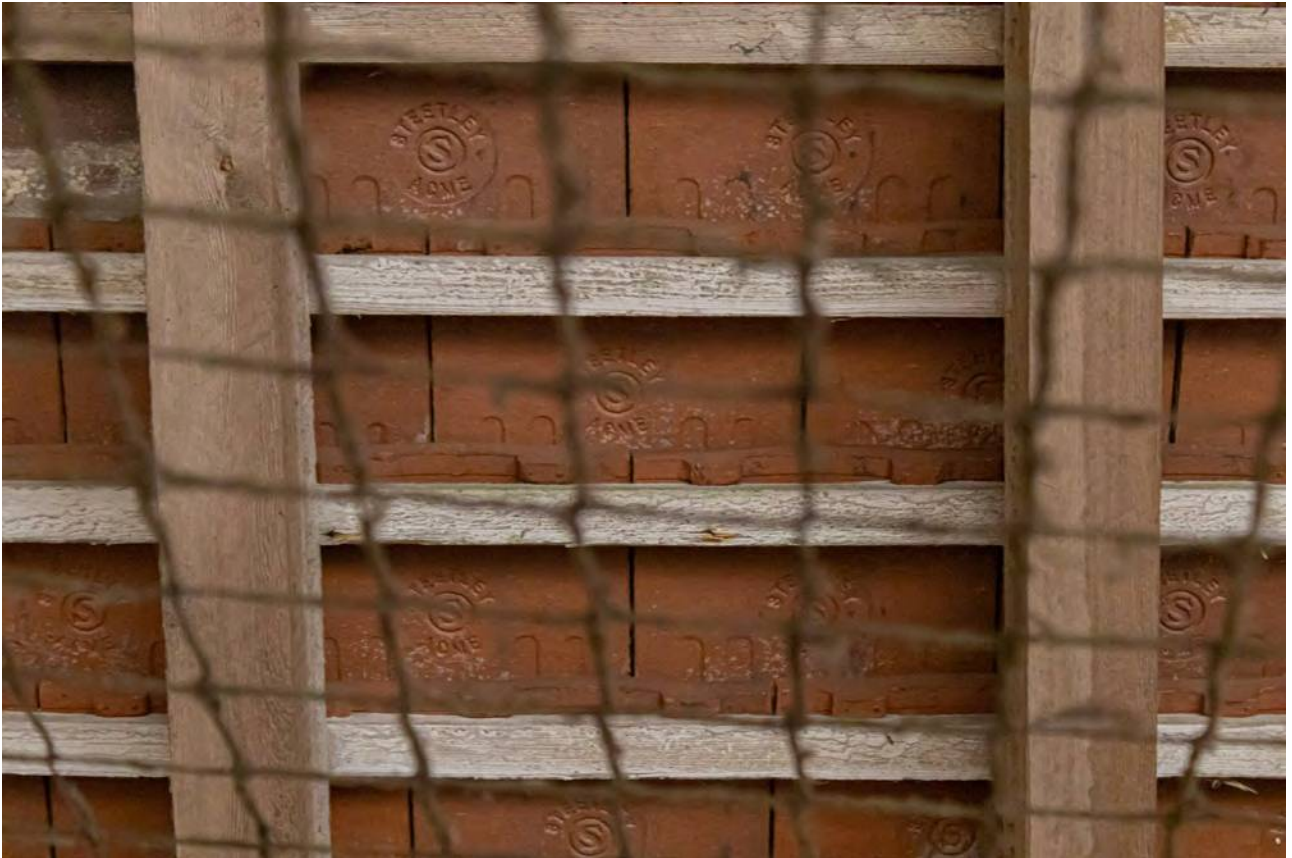
Plate 127 (127): Room 3, detail of underside of pantiles showing manufacturer's mark, from the north-west
