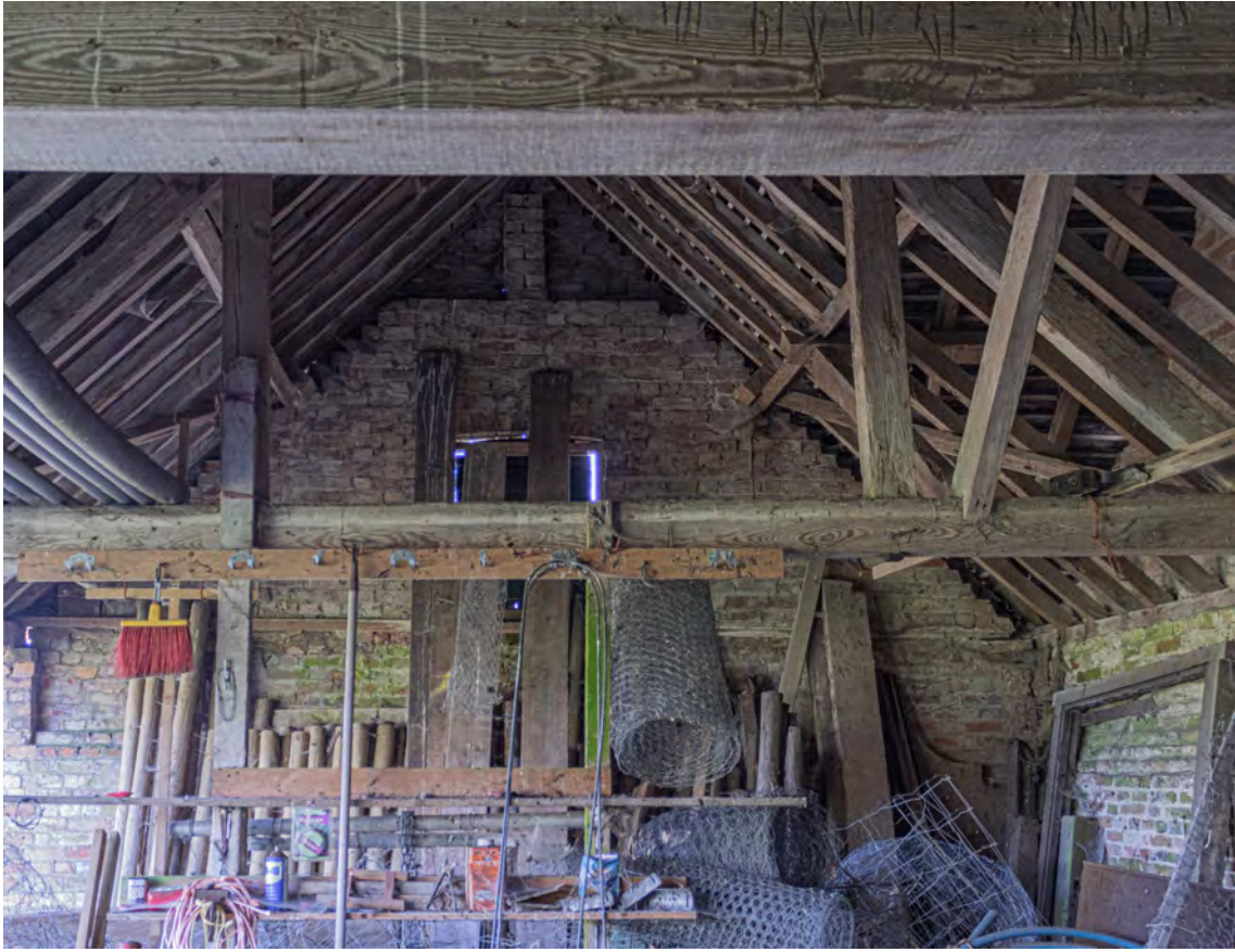
Plate 97 (090): Room 2, general view from the north-west
