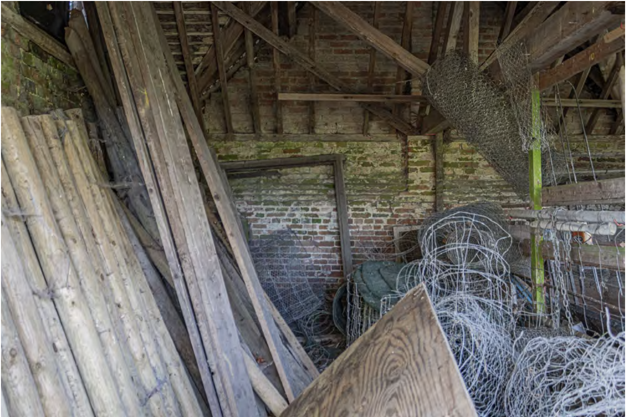
Plate 95 (102): Room 2, general view of the south-west wall [32], from the north-east
