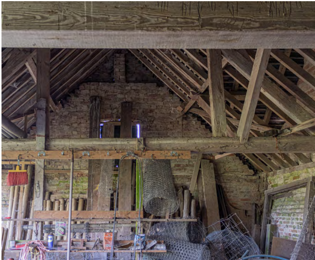
Plate 104 (090): Room 2, general view of Truss F, from the north-west
