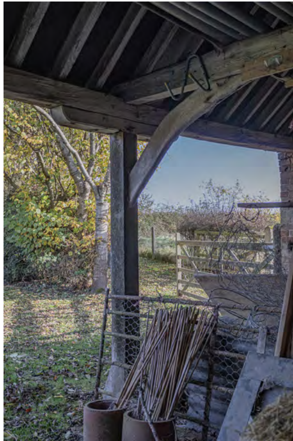
Plate 111 (096): Room 2, detail of post [19] in the north-east side and arched brace supporting Truss F, from the west
