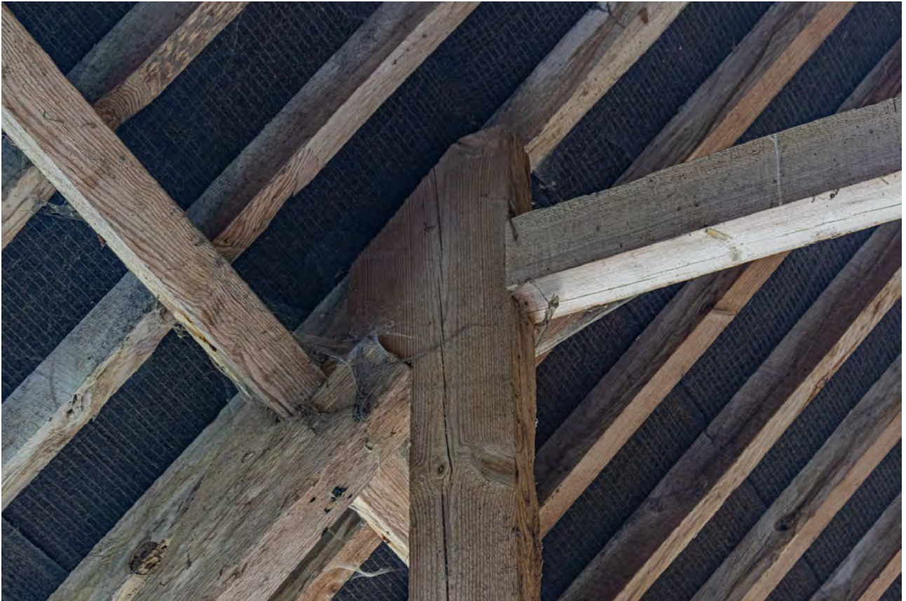
Plate 115 (095): Room 2, detail of top of Queen post connecting to the purlin beam in the south-west side of Truss D, from the SSE
