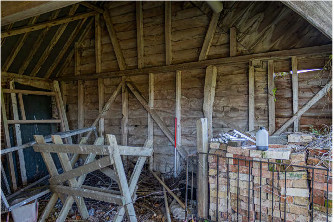
Plate 101 (087): Room 2, general view of the north-west wall [34] from the ESE
