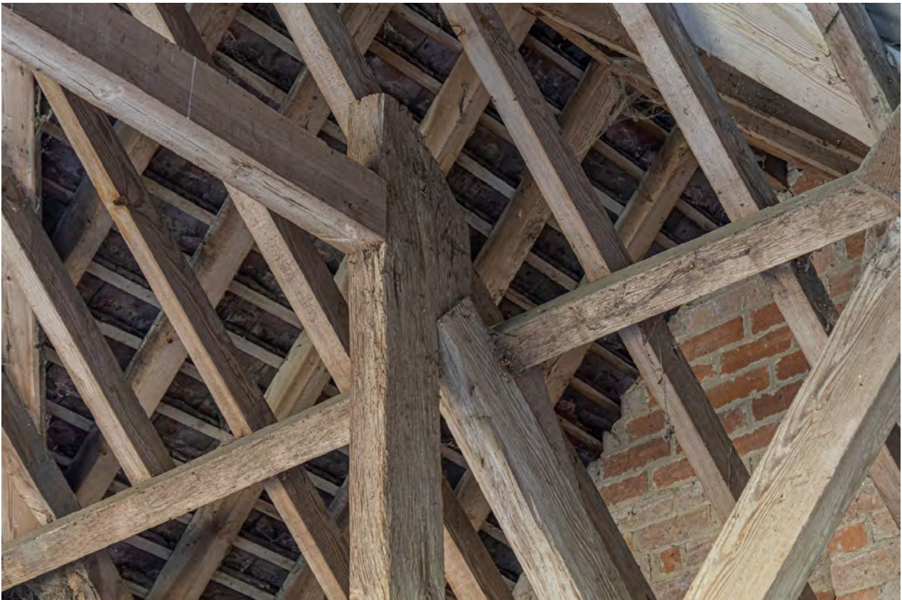
Plate 114 (094): Room 2, detail of top of Queen post connecting to the purlin beam in the south-west side of Truss F, from the NNE
