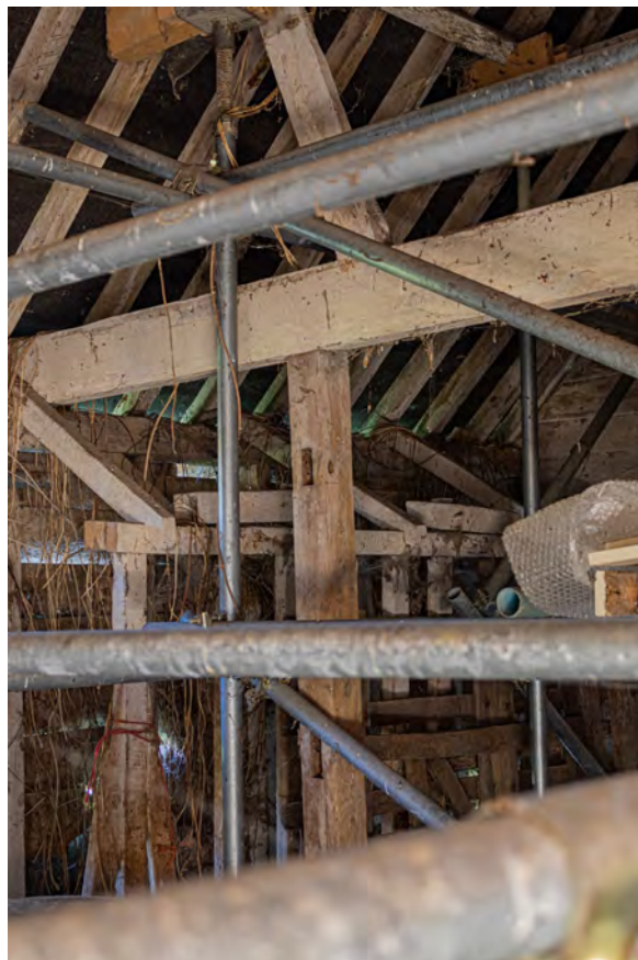
Plate 88 (113): Room 1, detail of post supporting the north-east side of the tie beam of Truss A to the north-east side, from the west
