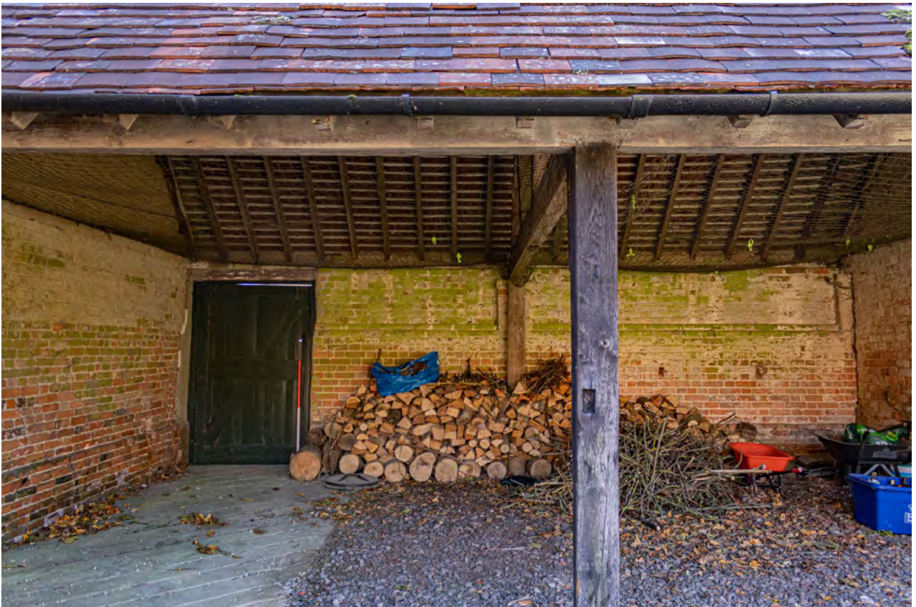
Plate 120 (075): Room 3, general view from the north-west
