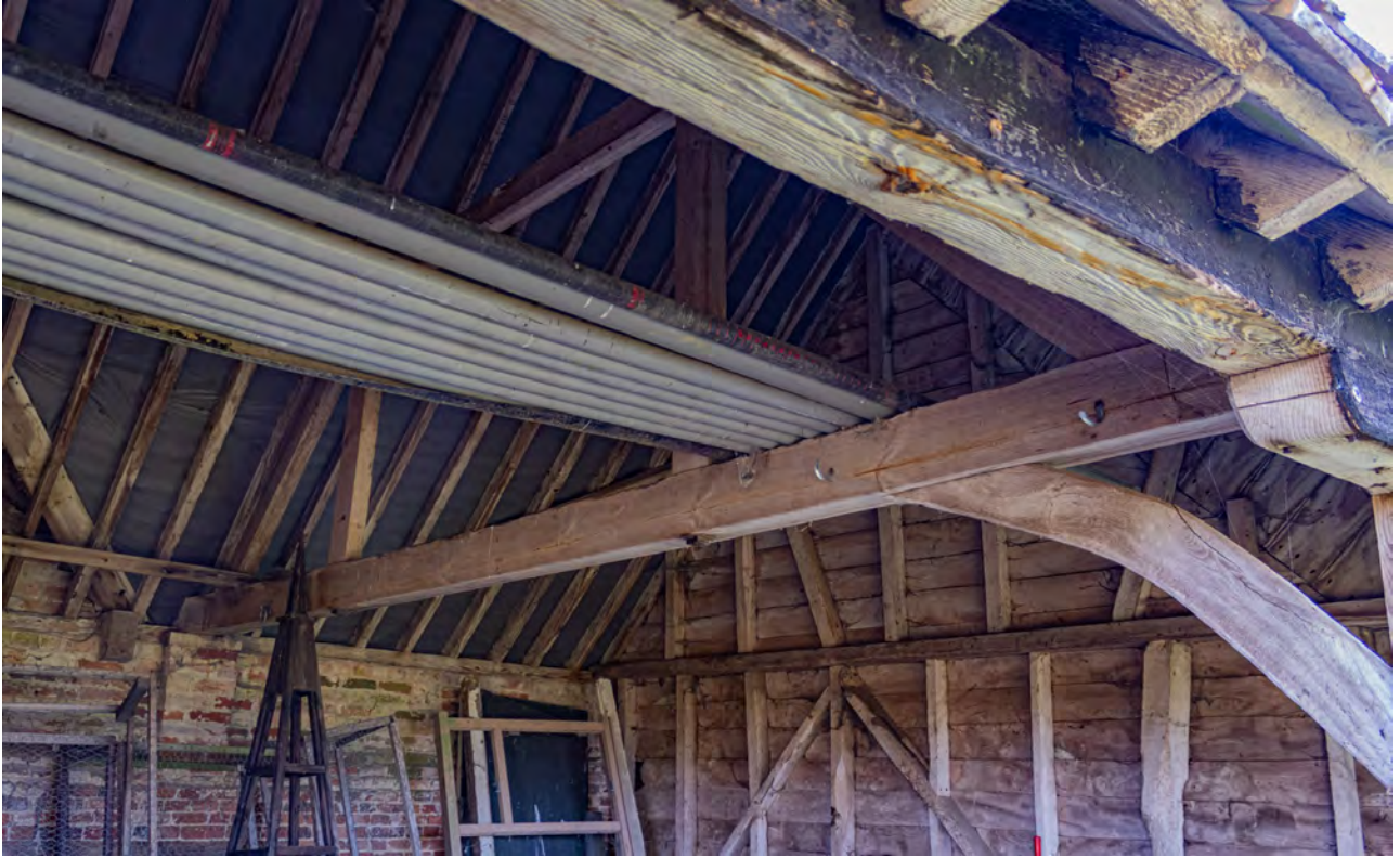
Plate 107 (099): Room 2, detail of Truss E from the ESE
