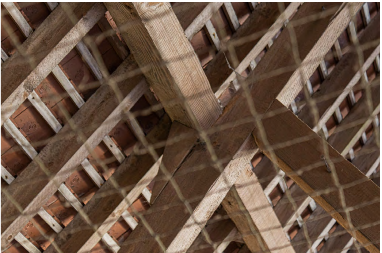
Plate 126 (084): Room 3, detail of purlin beam and rafter in the south-east side, from the north-east
