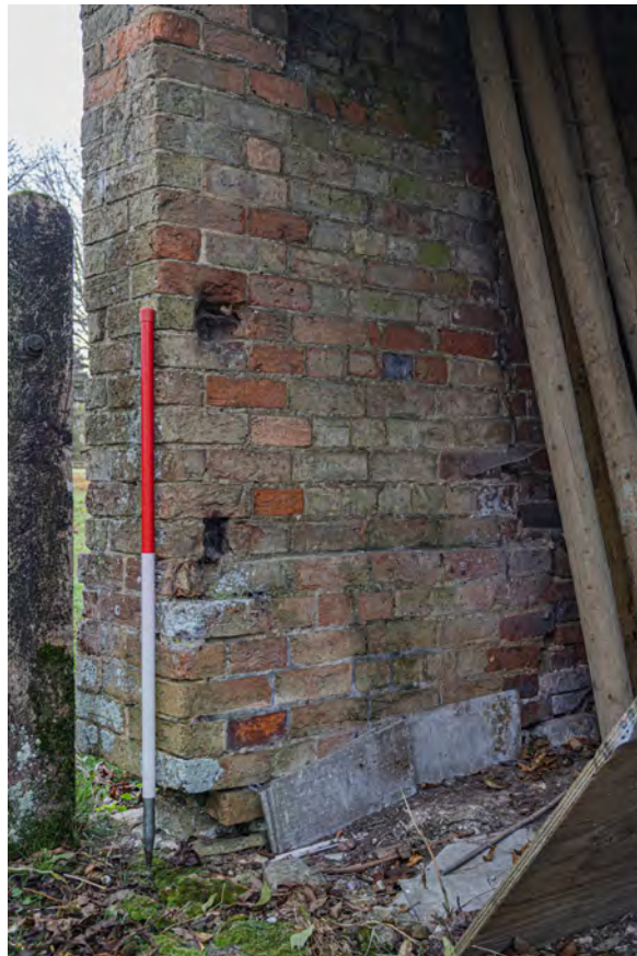
Plate 98 (043): Room 2, detail of slots in the north-east end of the south-east wall [33], from the north
