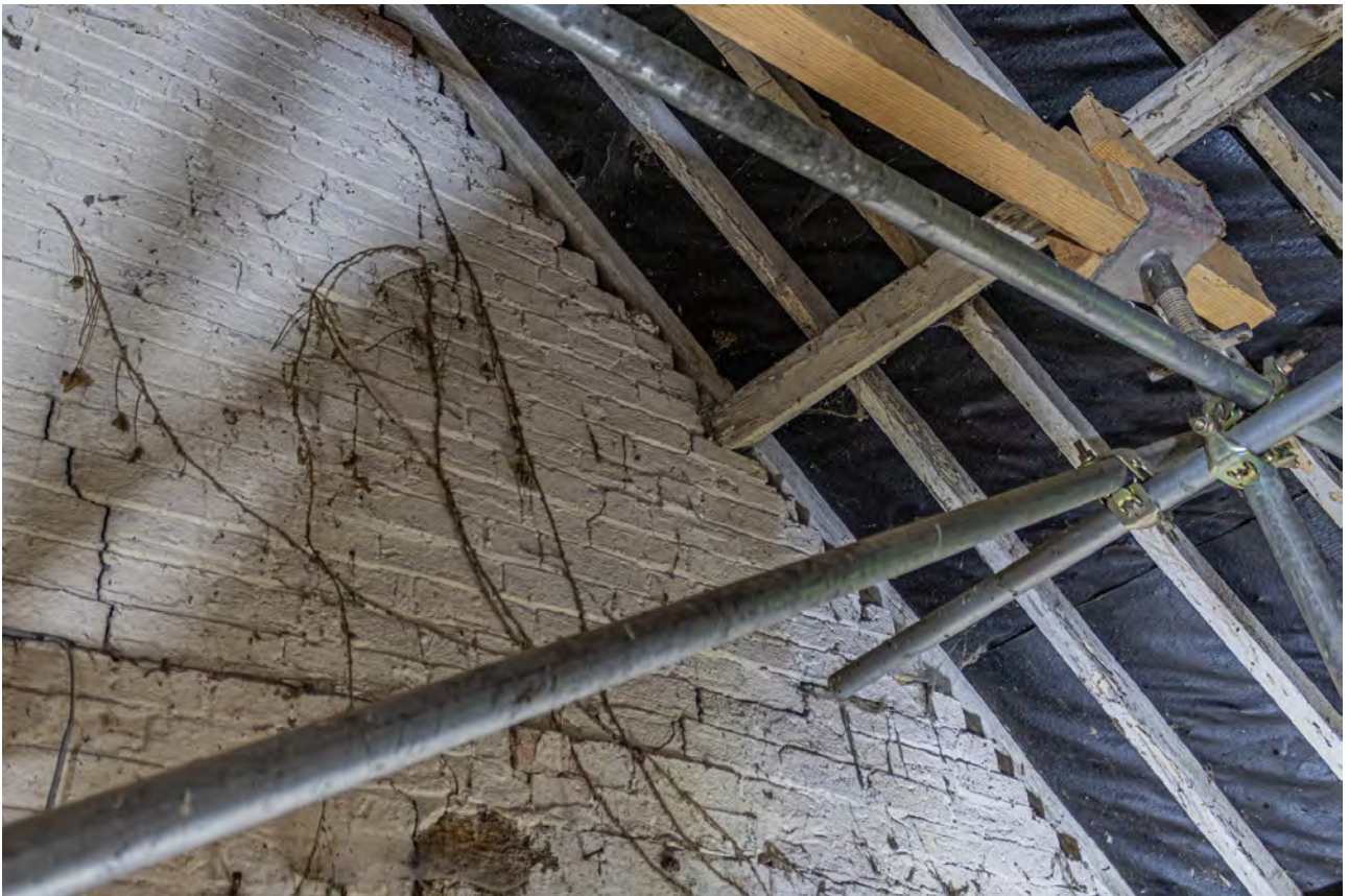
Plate 84 (055): Room 1, detail of the north-west gable wall [28] from the south-west
