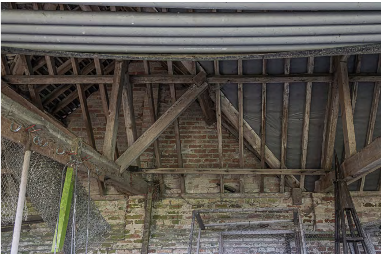
Plate 96 (100): Room 2, general view of the south-west wall [32], from the north-east
