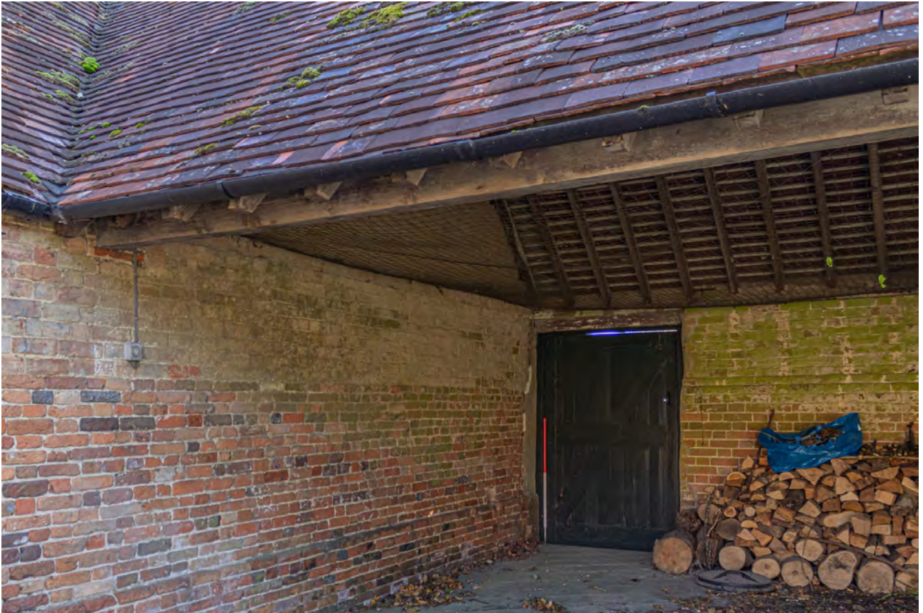
Plate 119 (076): Room 3, general view of the interior north-east wall, from the WNW
