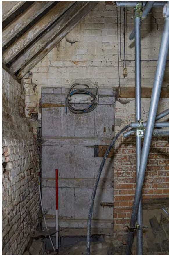
Plate 83 (053): Room 1, detail of door [31] in the north-west wall [28], from the south-east
