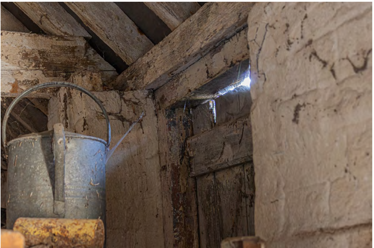
Plate 76 (062): Room 1, detail of opening [06] in the south-east side, from the north
