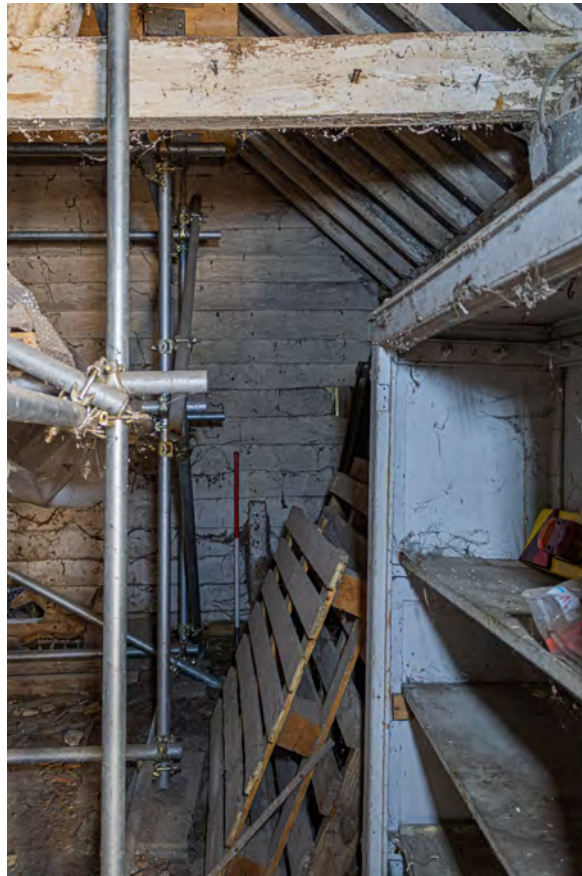
Plate 81 (063): Room 1, general view of wall [28] from the north-west
