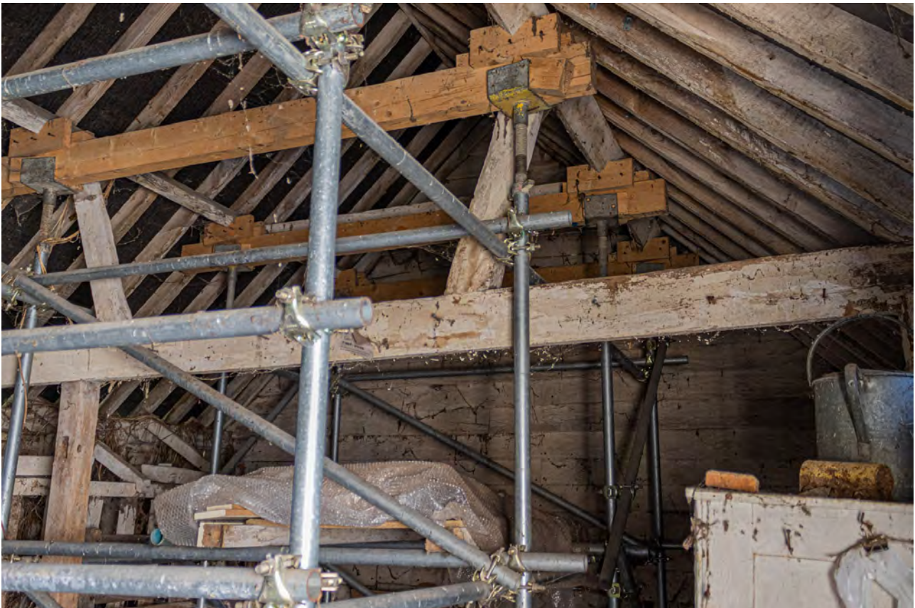
Plate 90 (065): Room 1, general view of Truss D from the WNW
