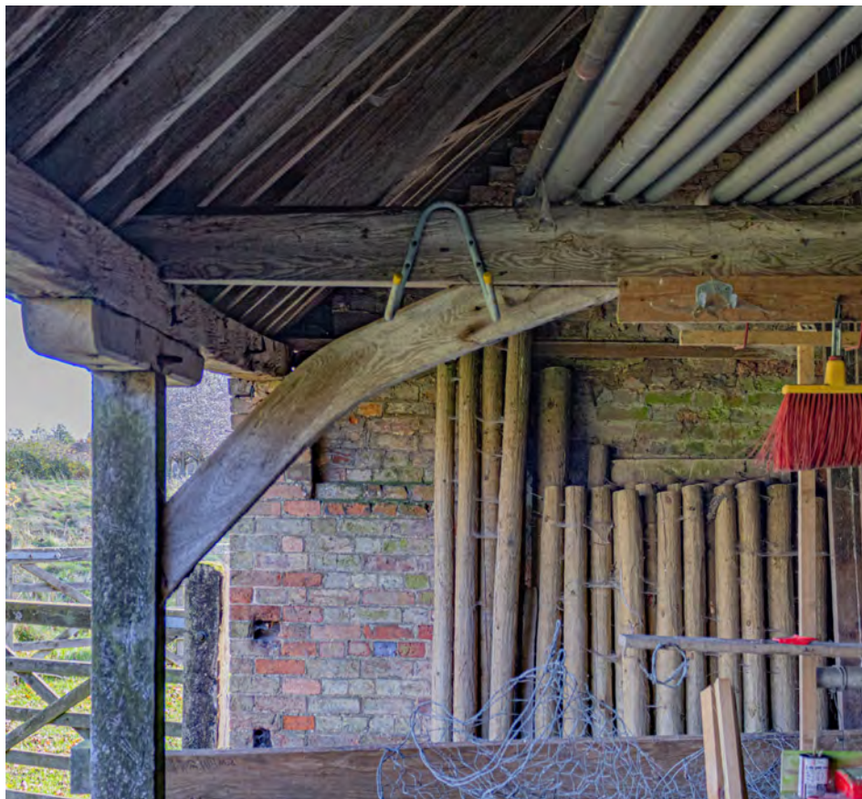
Plate 112 (097): Room 2, detail of post [19] in the north-east side and arched brace supporting Truss F, from the north-west
