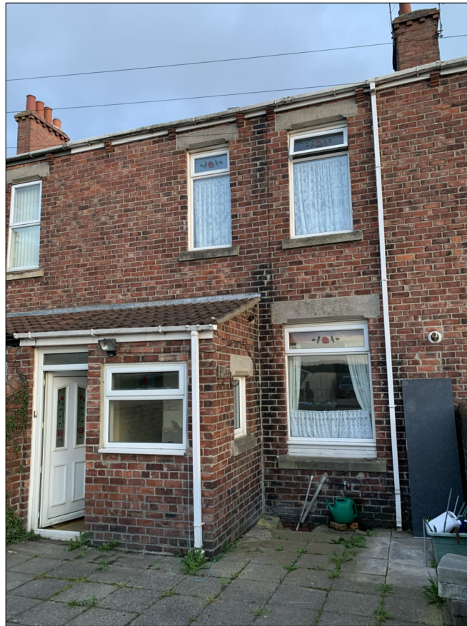
Photo 2 : View of rear of No 34 as from inside of rear yard.
