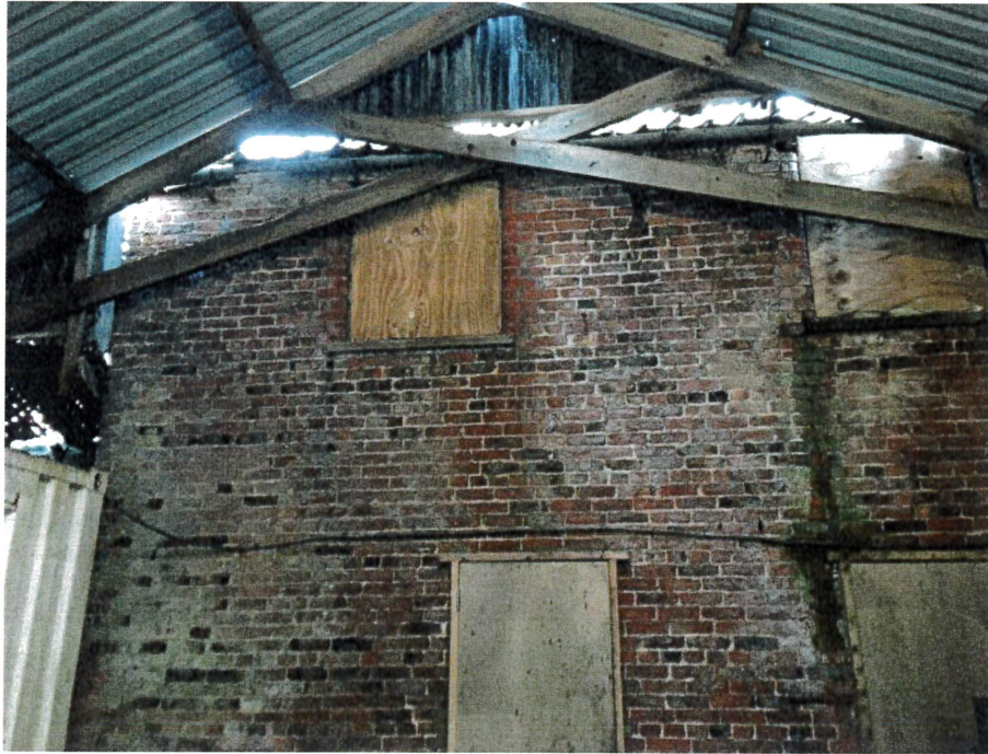
Rear Of Northern Barn Showing Infill Section
