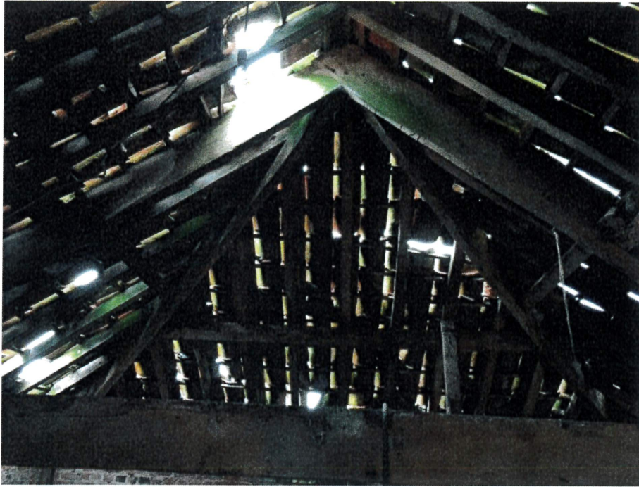
Trusses and Roof Covering North Barn
